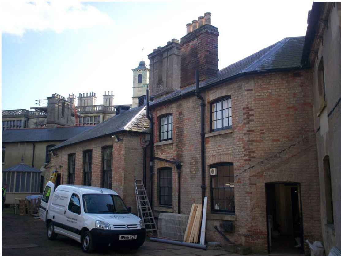
Plate 4: External view of wet laundry (view
