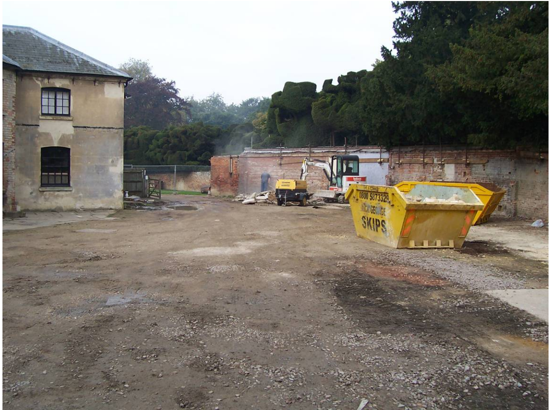
Plate 1: General view of service yard prior to works
