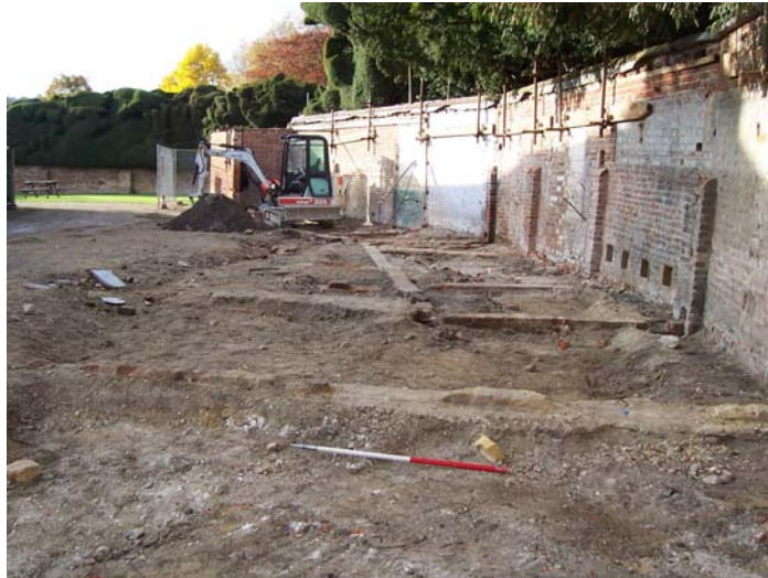
General view of remains of service yard outbuildings. (1m scale).
