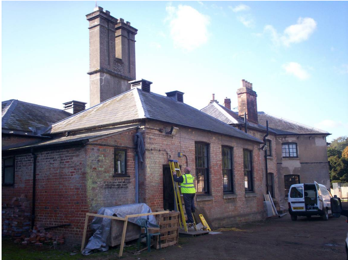
Plate 3: External view of wet laundry (view )
