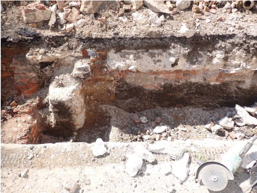
Photograph 4: South end of the trench, east-facing section
