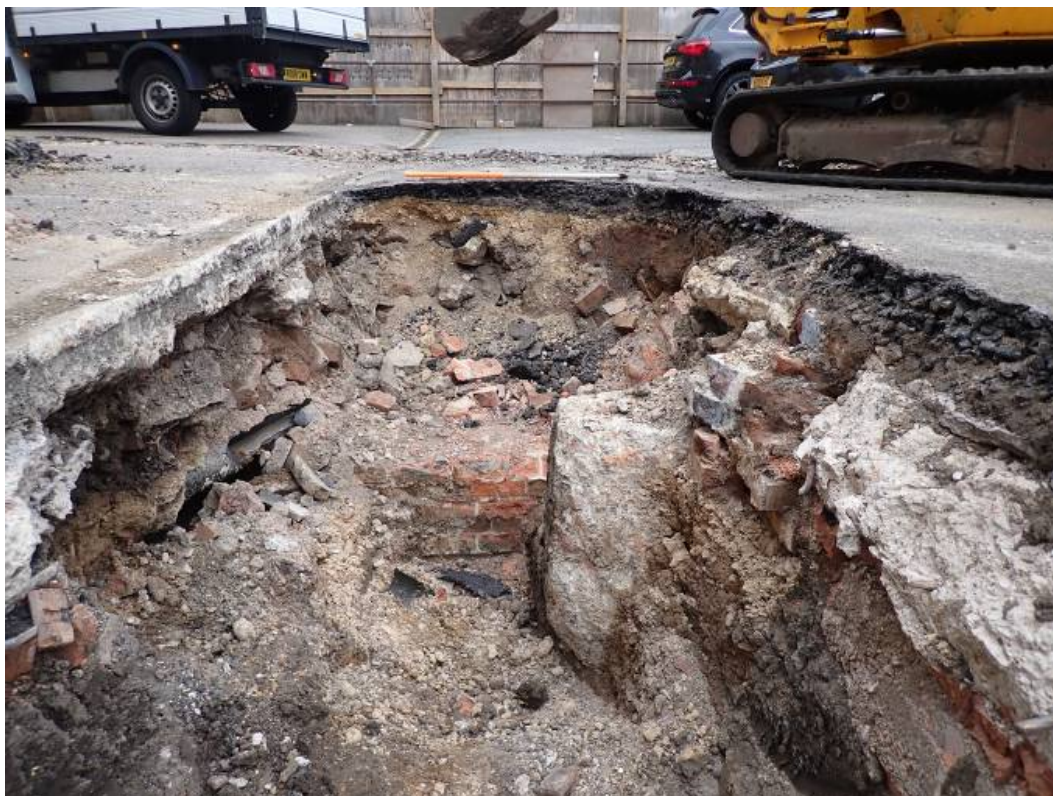
Photograph 6: Looking towards the south end of the trench (scale 1m)
