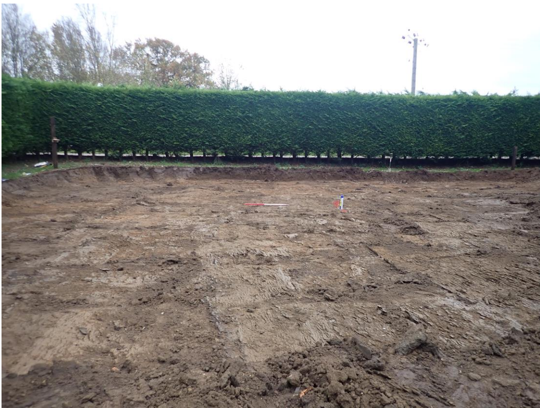
Area of ground reduction, looking south
