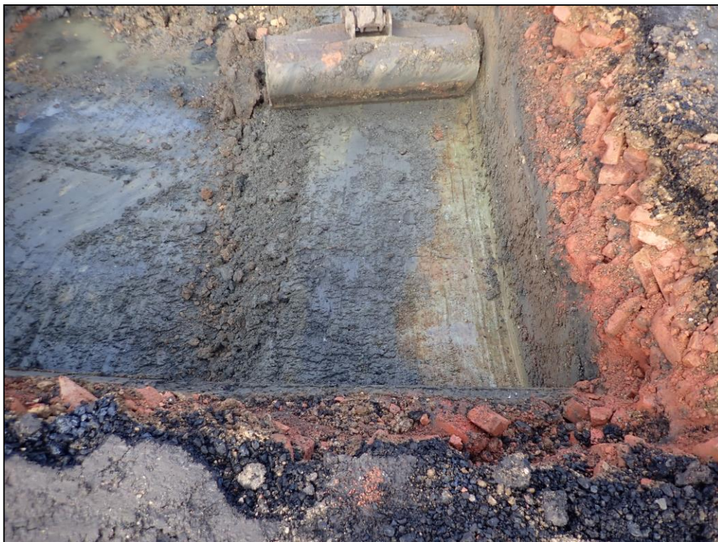
Figure 4: Trench 2 during machine excavation, palaeochannel [205] visible to left of image Looking north-west.
