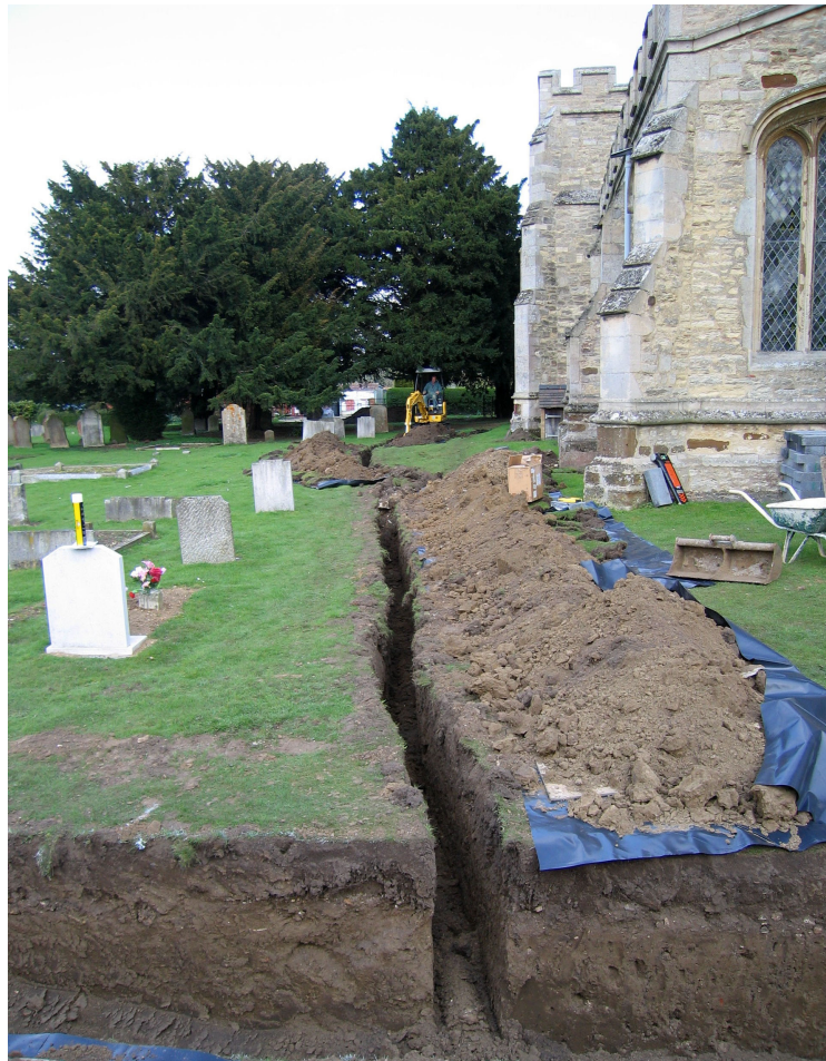
Excavation in progress north of the church
