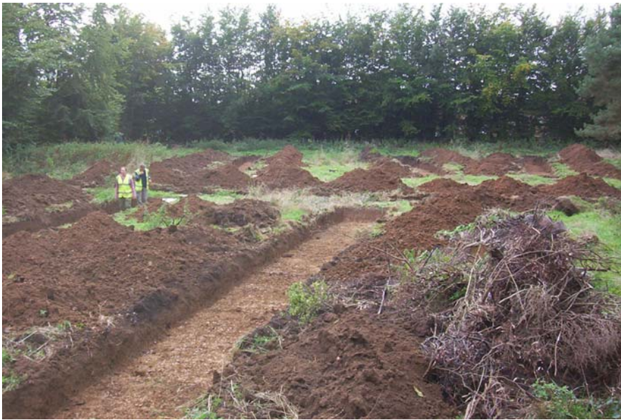
Trench 5, looking south-west.
