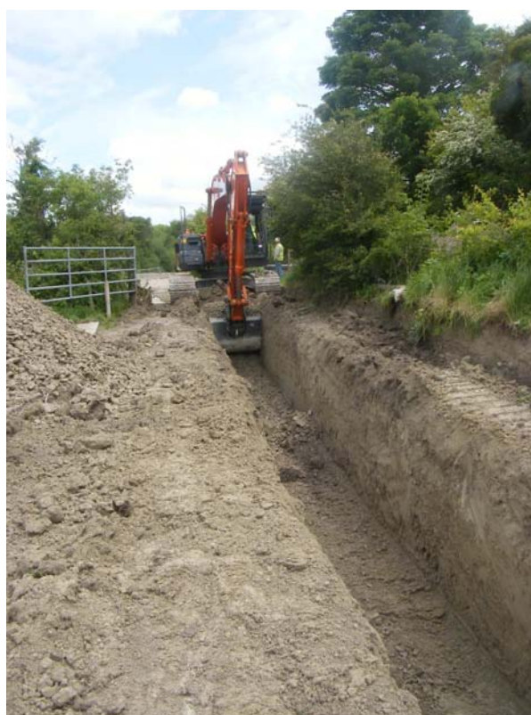
Plate 2: Excavation of pipe trench above Sherrell Spring
