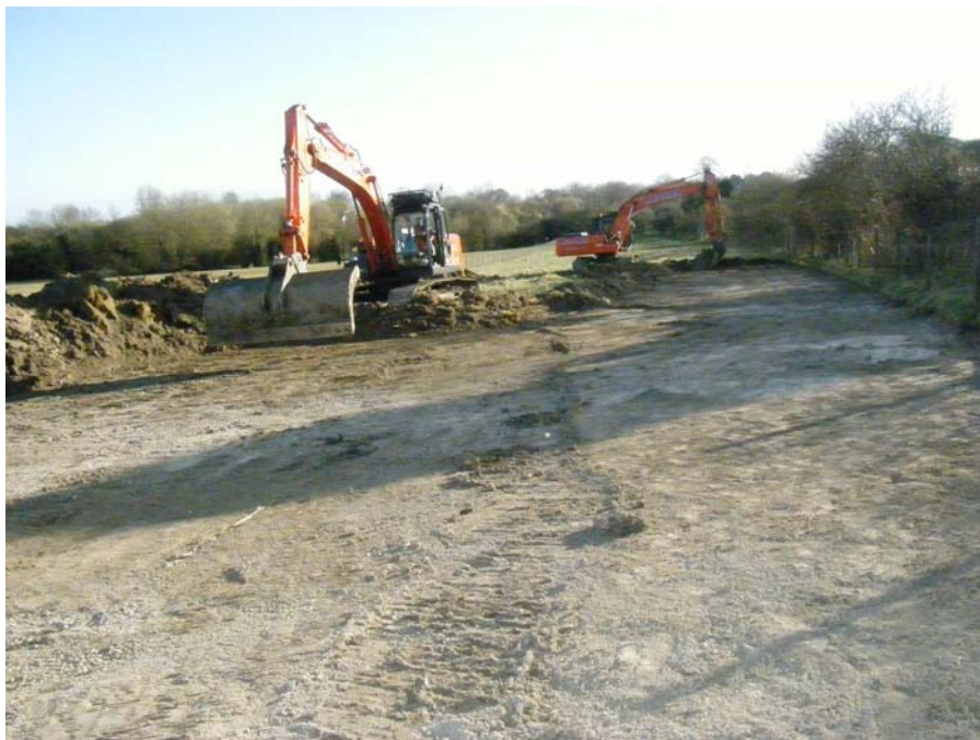
Plate 1: Stripping of topsoil from pipeline easement
