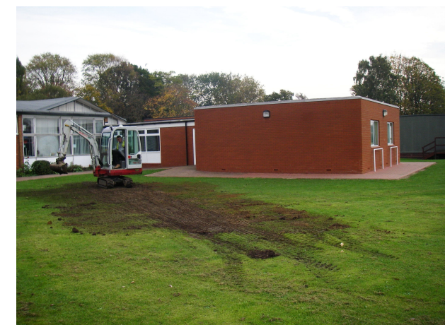
After backfilling. Looking south-east.
