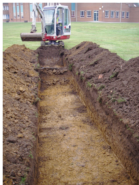
Stripping. Looking east.
