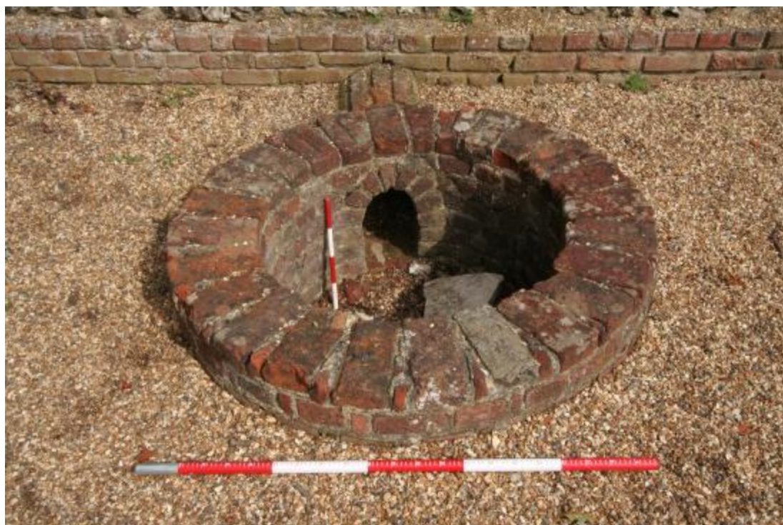
Plate 1: Area 1, well and culvert
