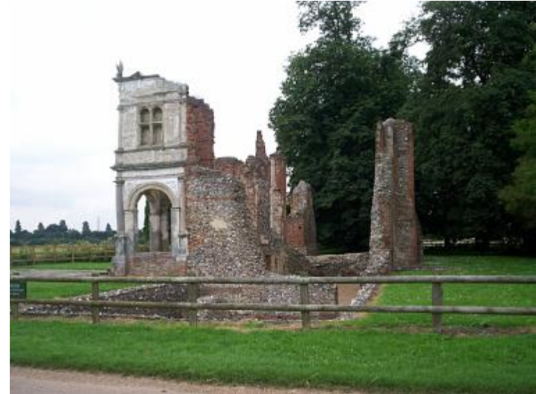
View from the north-east
