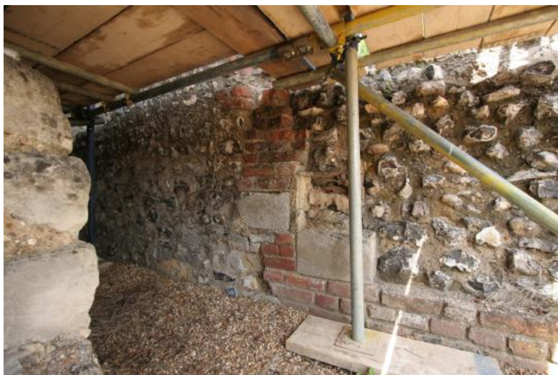
Plate 2: Area 1, masonry at the junction of the Hall and Area 1
