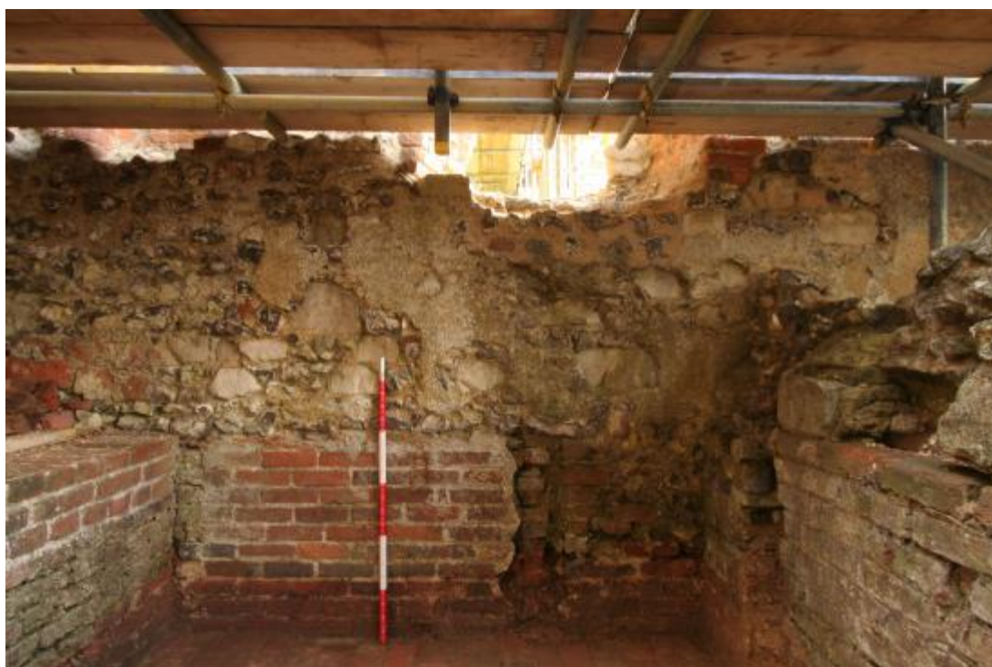
Plate 4: Area 3, looking east
