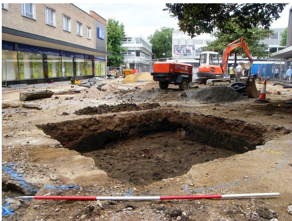
Site photograph. Looking west, Pit 6 in foreground. Scale 2m
