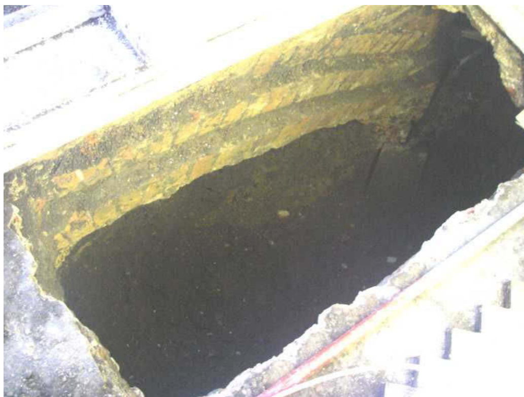
Figure 5: Trench 2 relieving arch of post-medieval wall foundation
