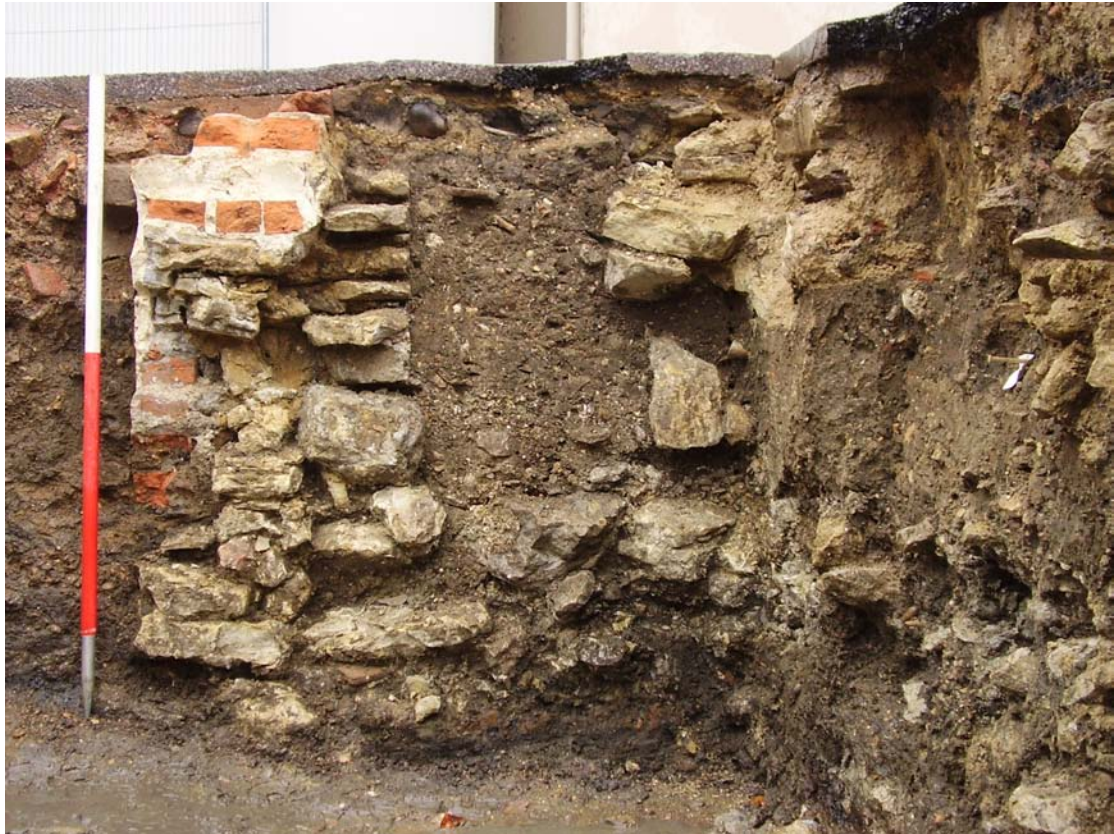
Figure 19: Culvert in north-eastern corner of Test Pit 2 (Viewed from the south. Scale 1m)
