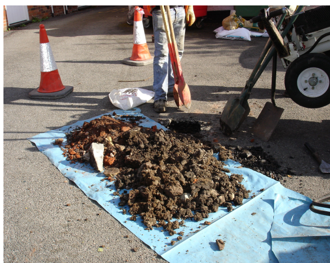
Spoil from the hand-excavated part of BH4 laid out for checking.
