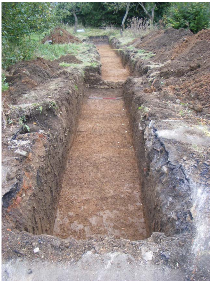
Plate 3: Trench 2, view from the north.
