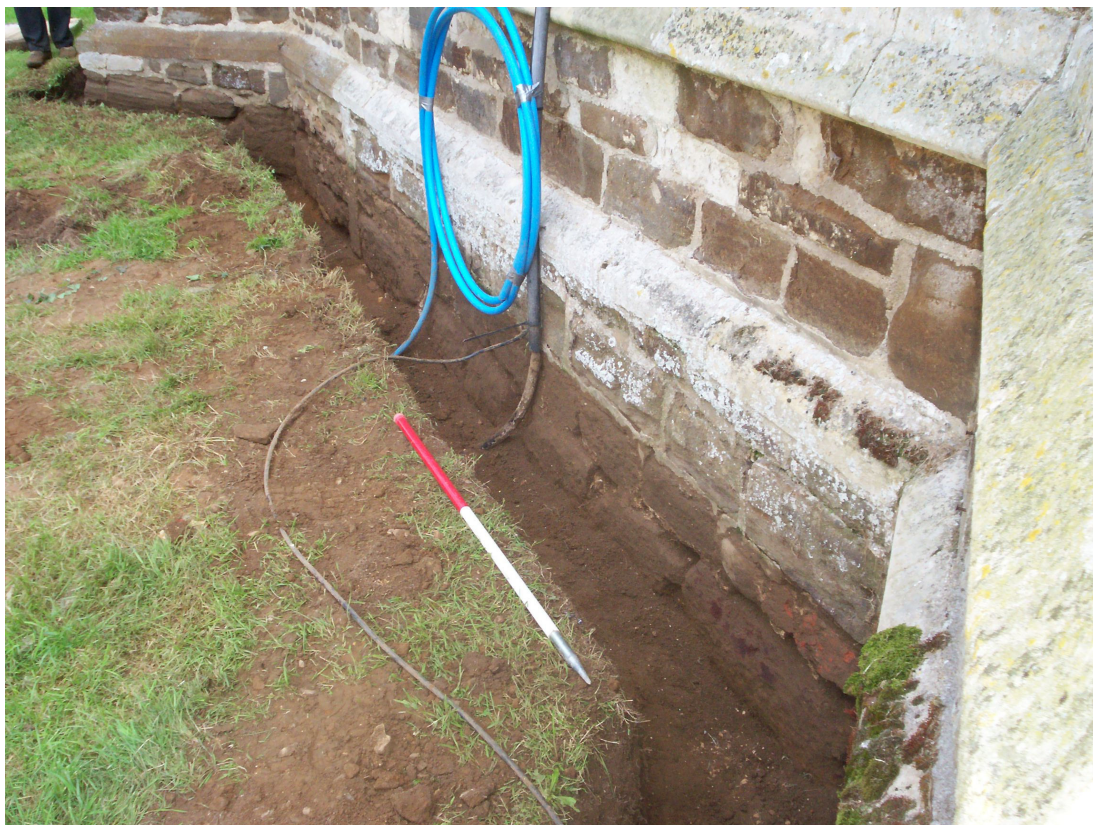
Figure 4: Excavations for French drain adjacent to west wall of tower
