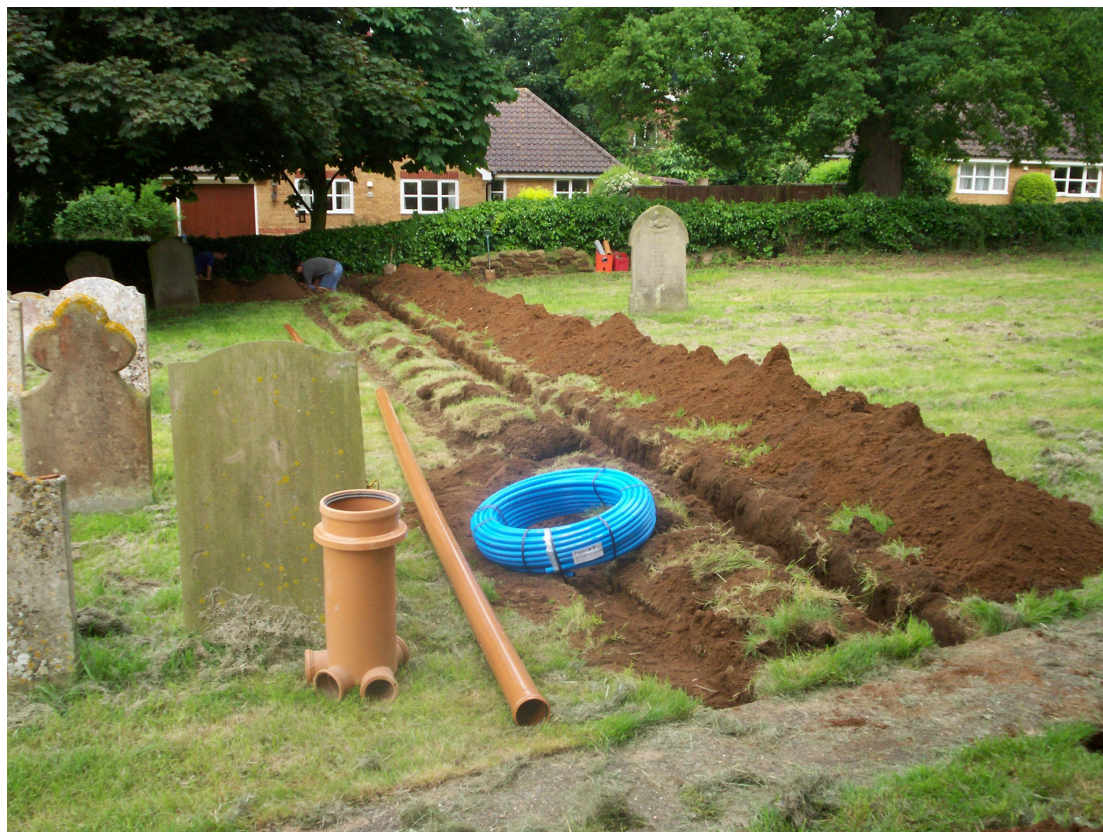
Figure 6: Excavations for soil pipe viewed from the tower.
