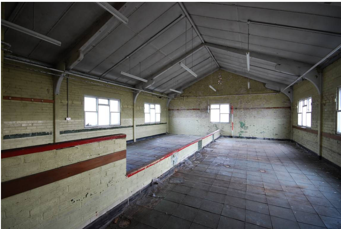
b) Shifting house (SPA1 administration)
