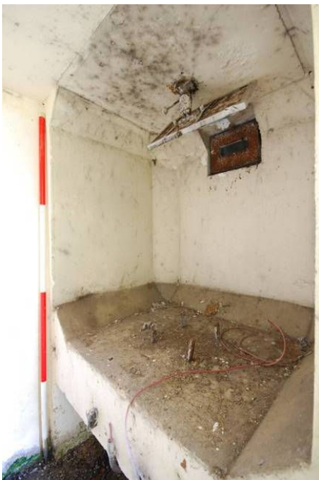
b) SPA45 (igniter testing) interior
