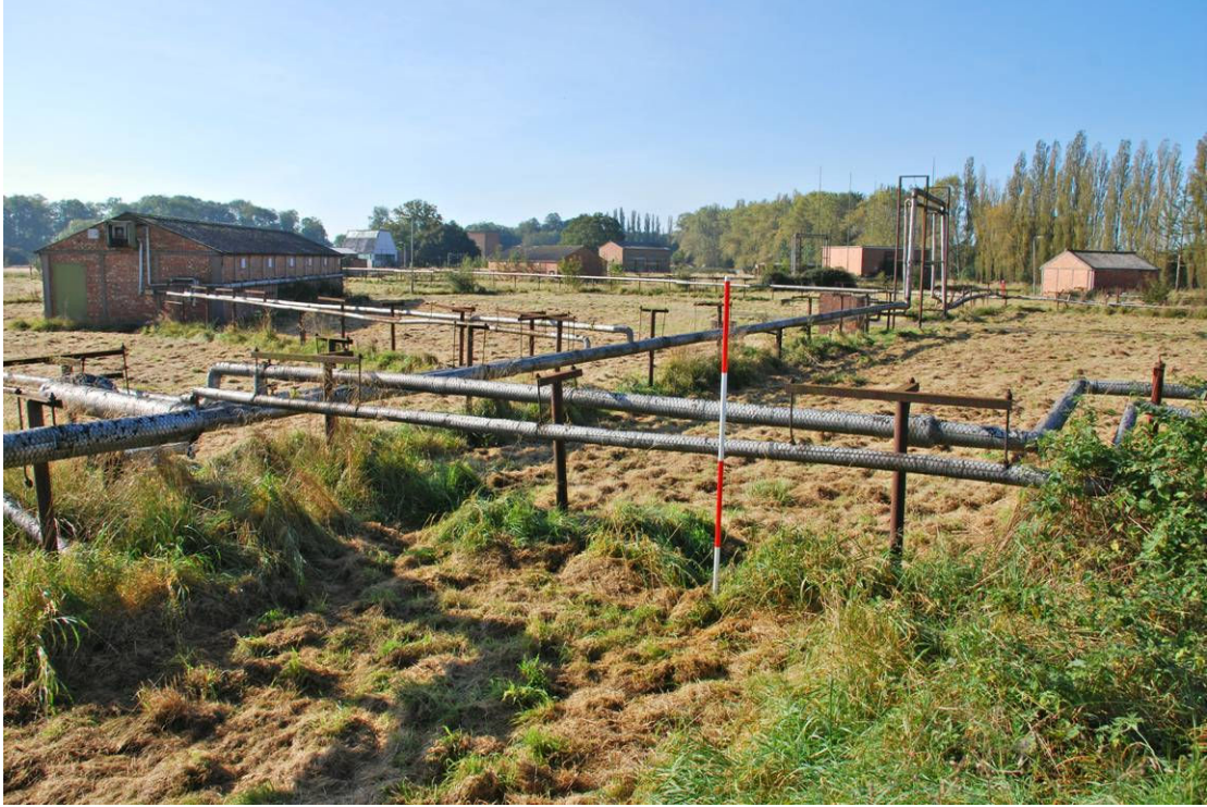
a) General view to show steam heating pipes
