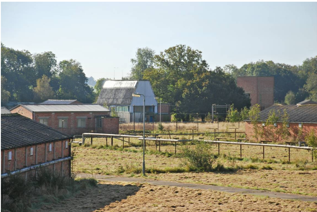
b) General view of Solids Area (view towards south)
