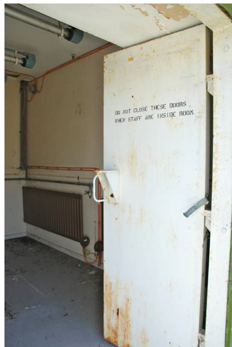
b) SPA42 (abrasive cutting) view into gable-end room
