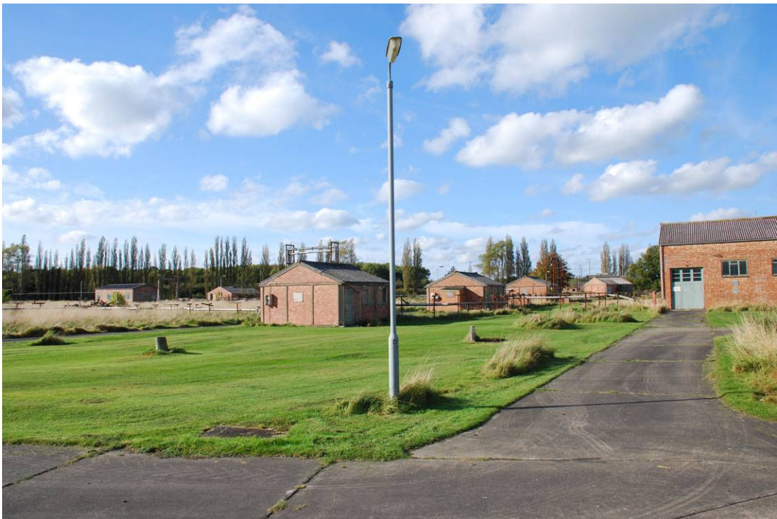
b) General view of Solids Area (view towards north)
