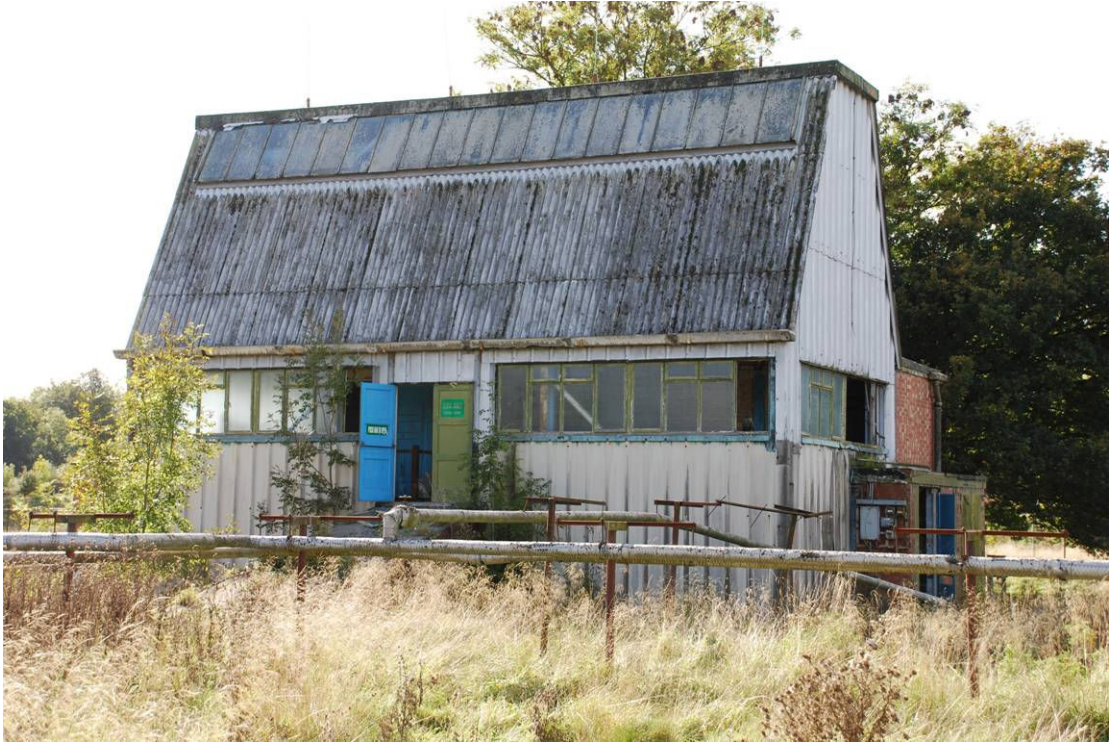
a) SPA37 (coating and tape winding)
