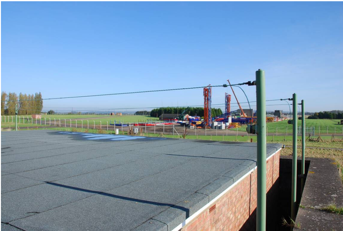
b) SPA21 (rocket motor magazine) lightning protection
