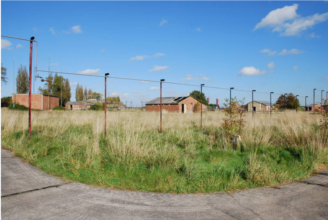
a) General view of Solids Area (view towards east)
