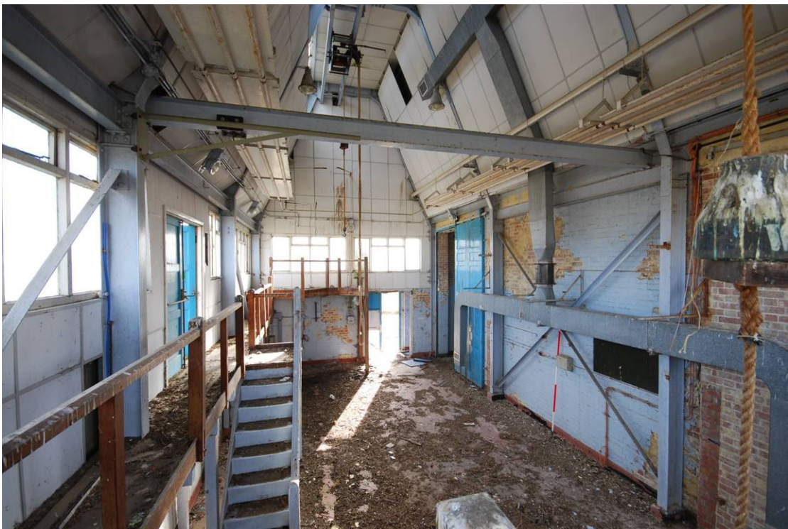
b) SPA37 (coating and tape winding) interior, main compartment
