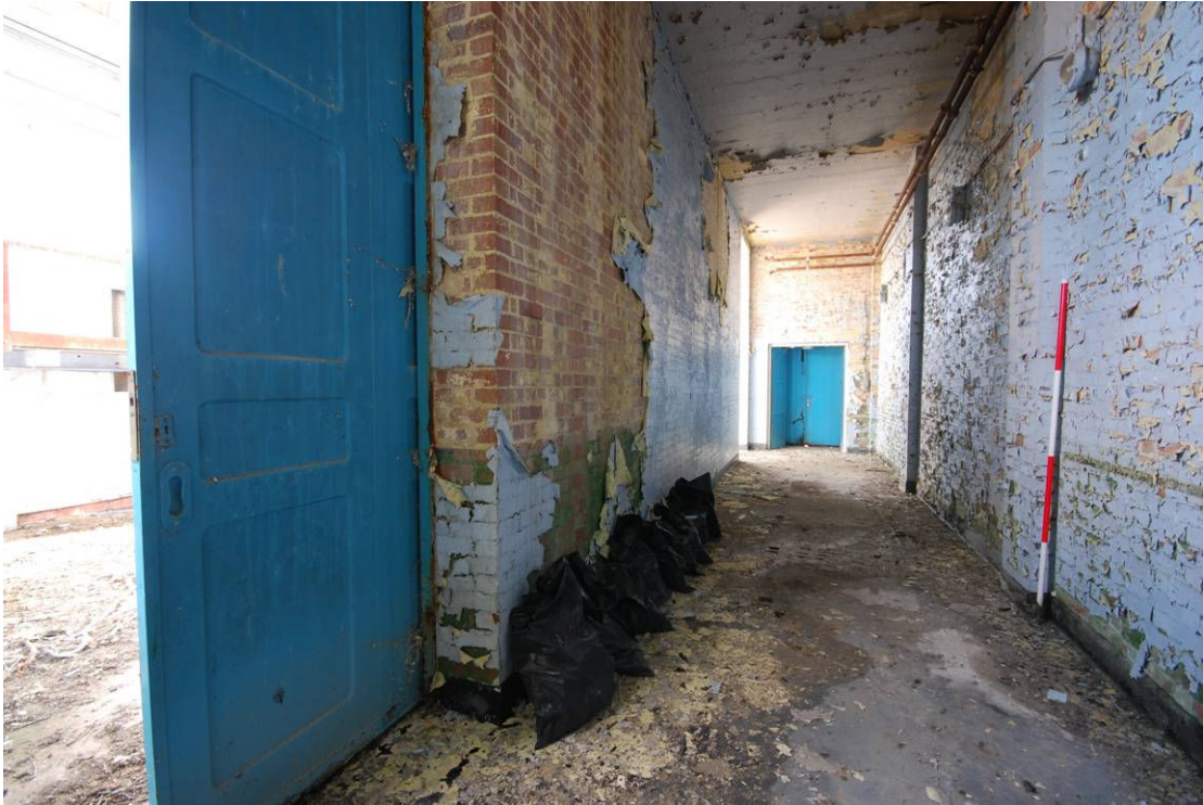
a) SPA37 (coating and tape winding) interior
