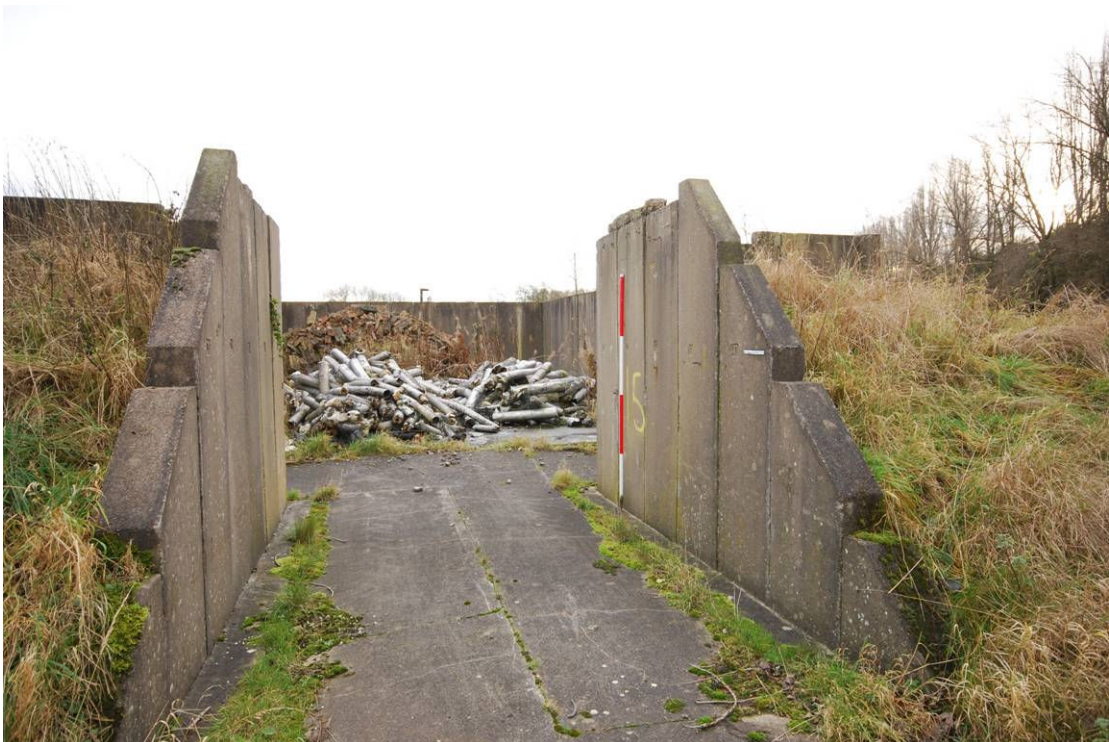
b) SPA15 (press) building demolished, traverse and concrete blast walls remain
