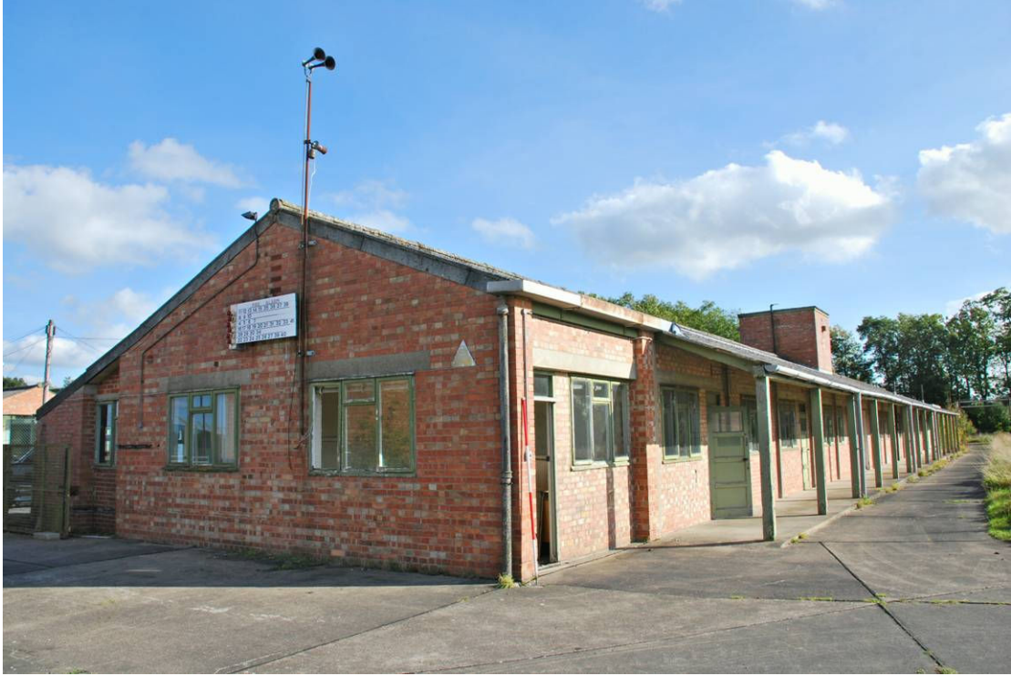
a) SPA1 Administration block
