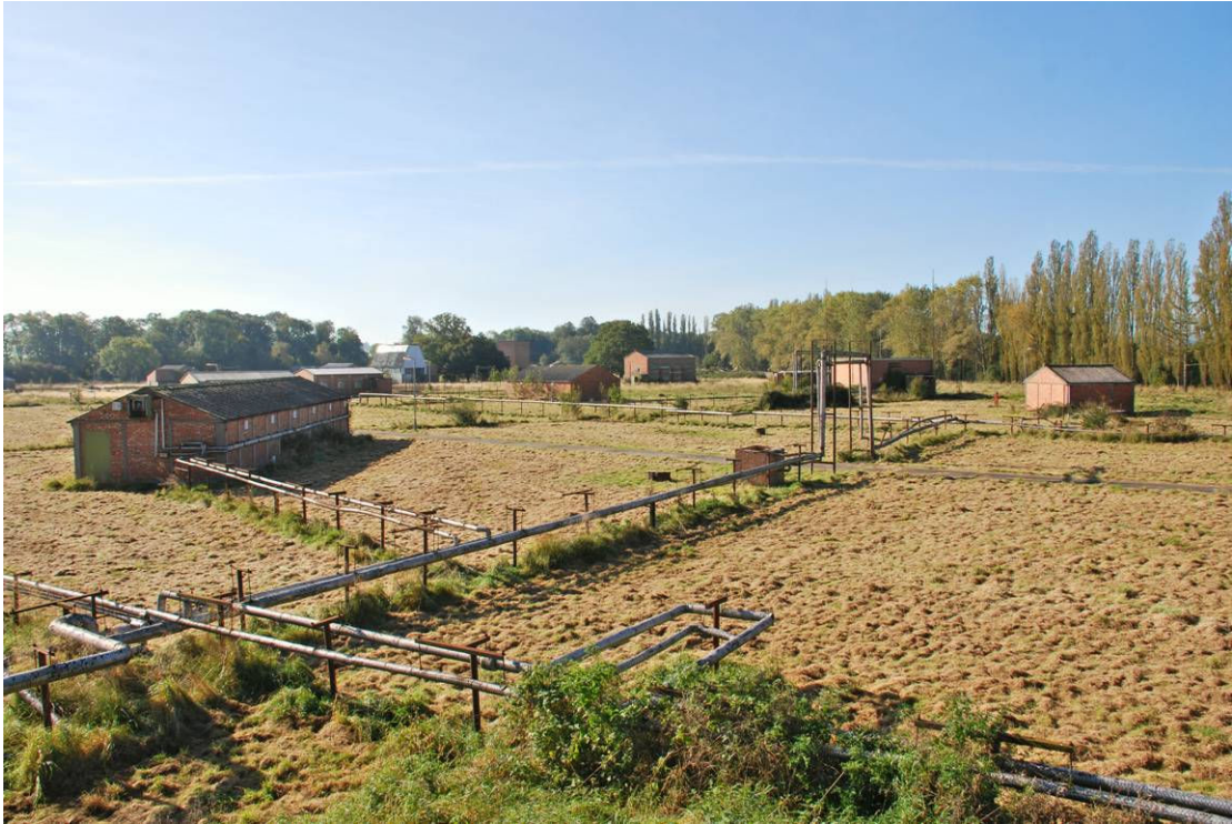
a) General view of Solids Area (view towards south west)
