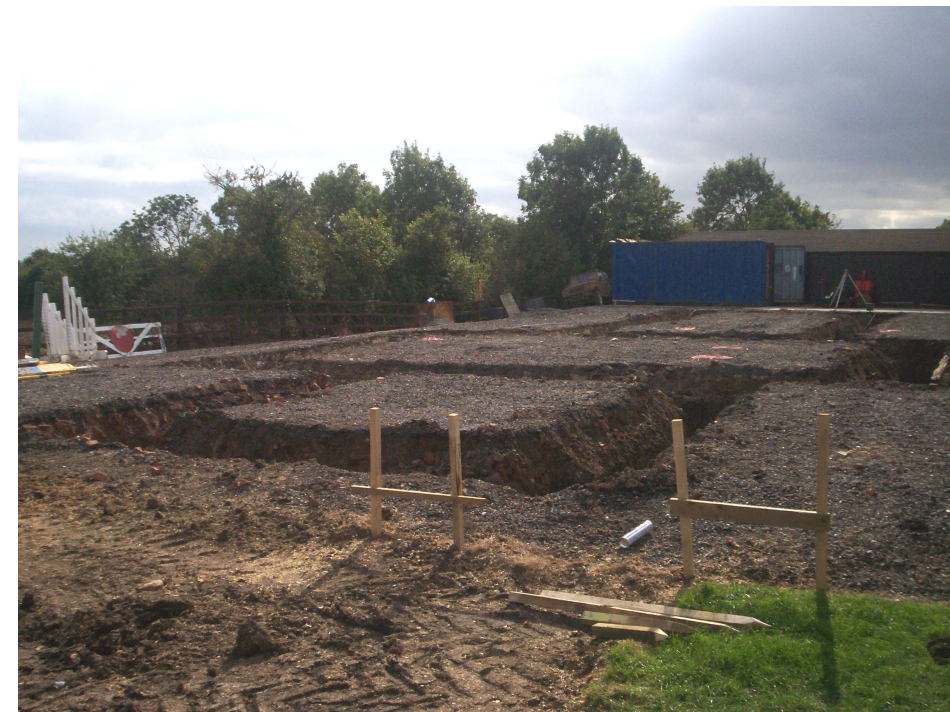
Foundation trench, looking south west.
