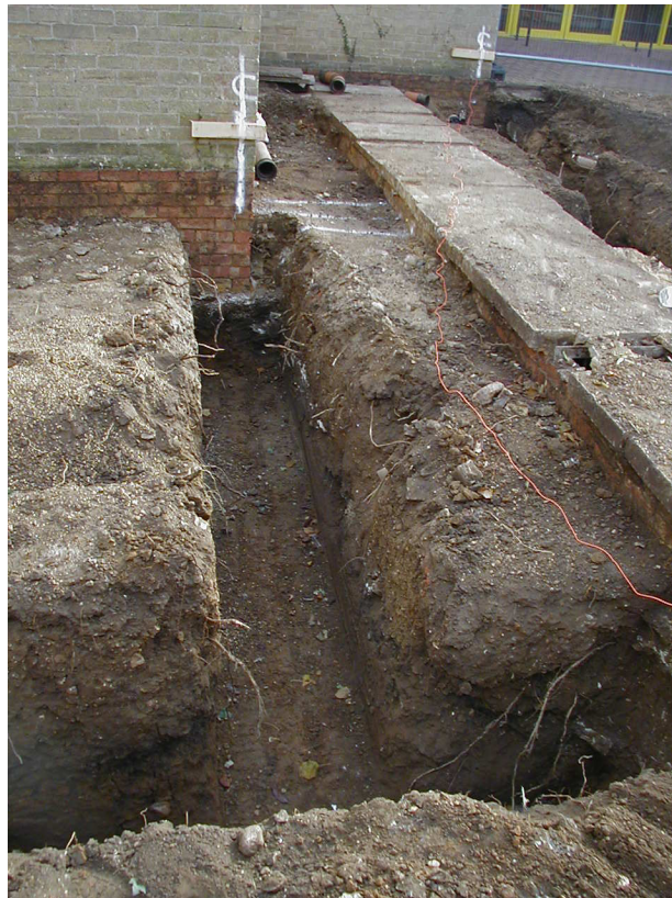
Plate 1: Footings facing east.
