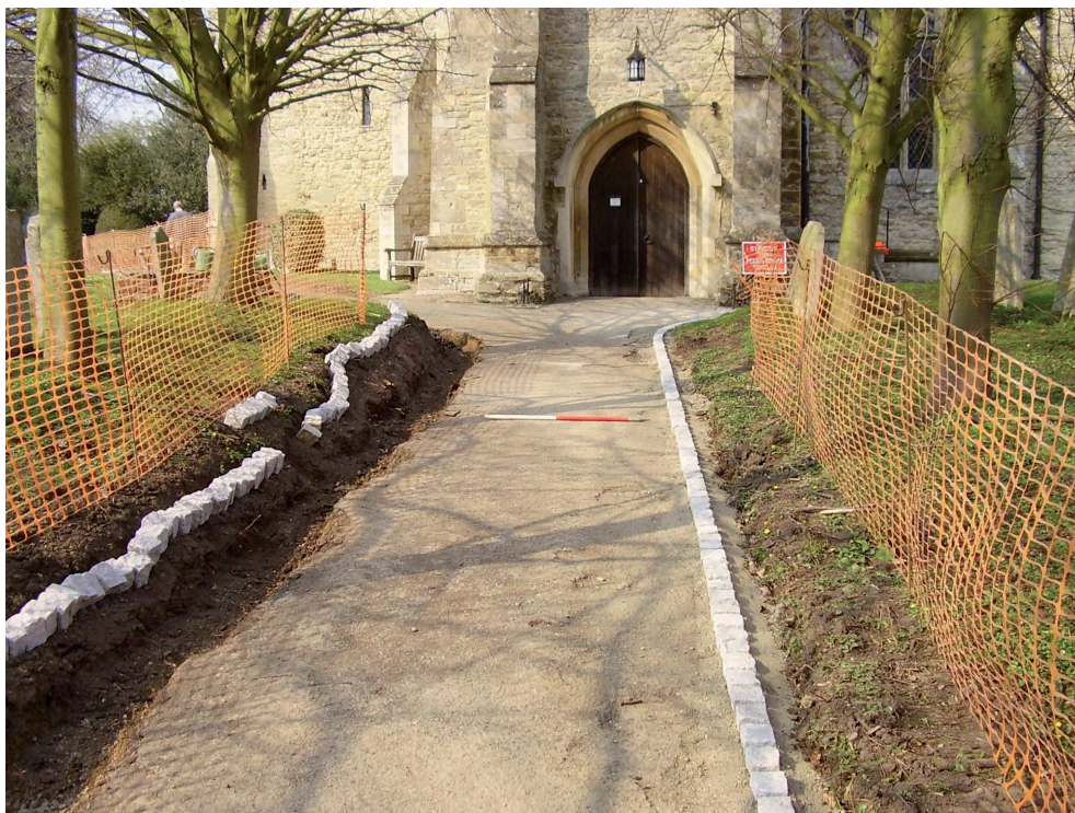
Plate 3: The trench for path edging stones. Looking north, scale 1m.
