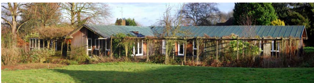
Plate 1: Western side of building
