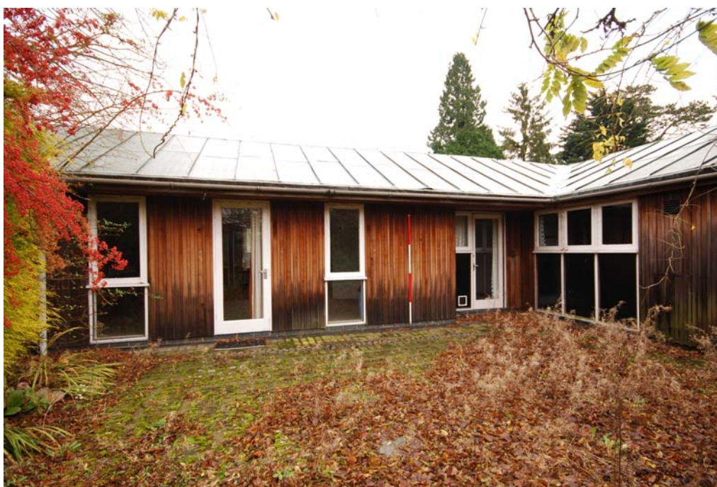
Plate 2: North wing and cross wing from courtyard at north-west of building
