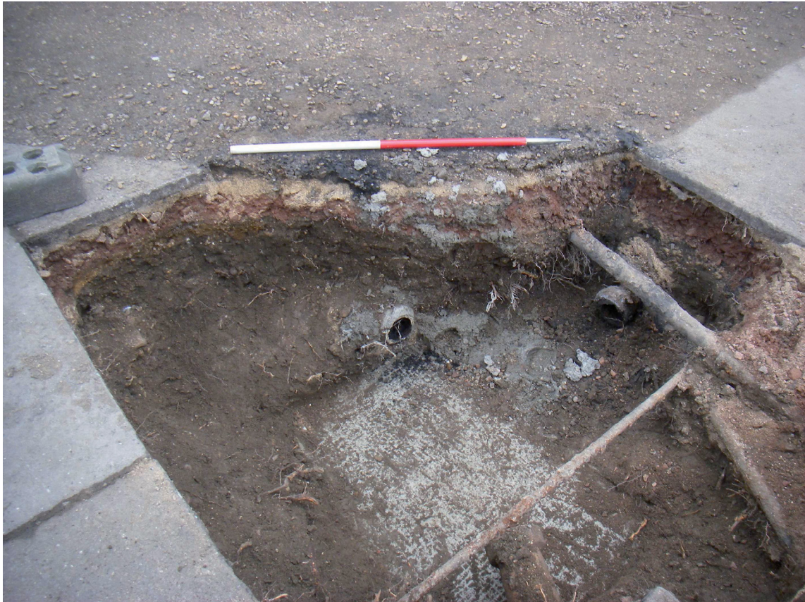
9. West End: Excavation for inspection chamber
