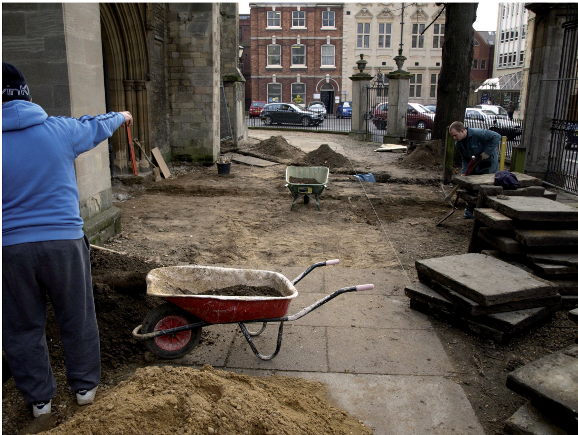
5. West End: Removal of paving slabs
