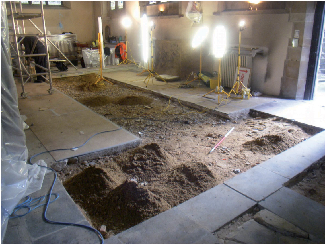
4. Trinity Chapel: Tiling removed
