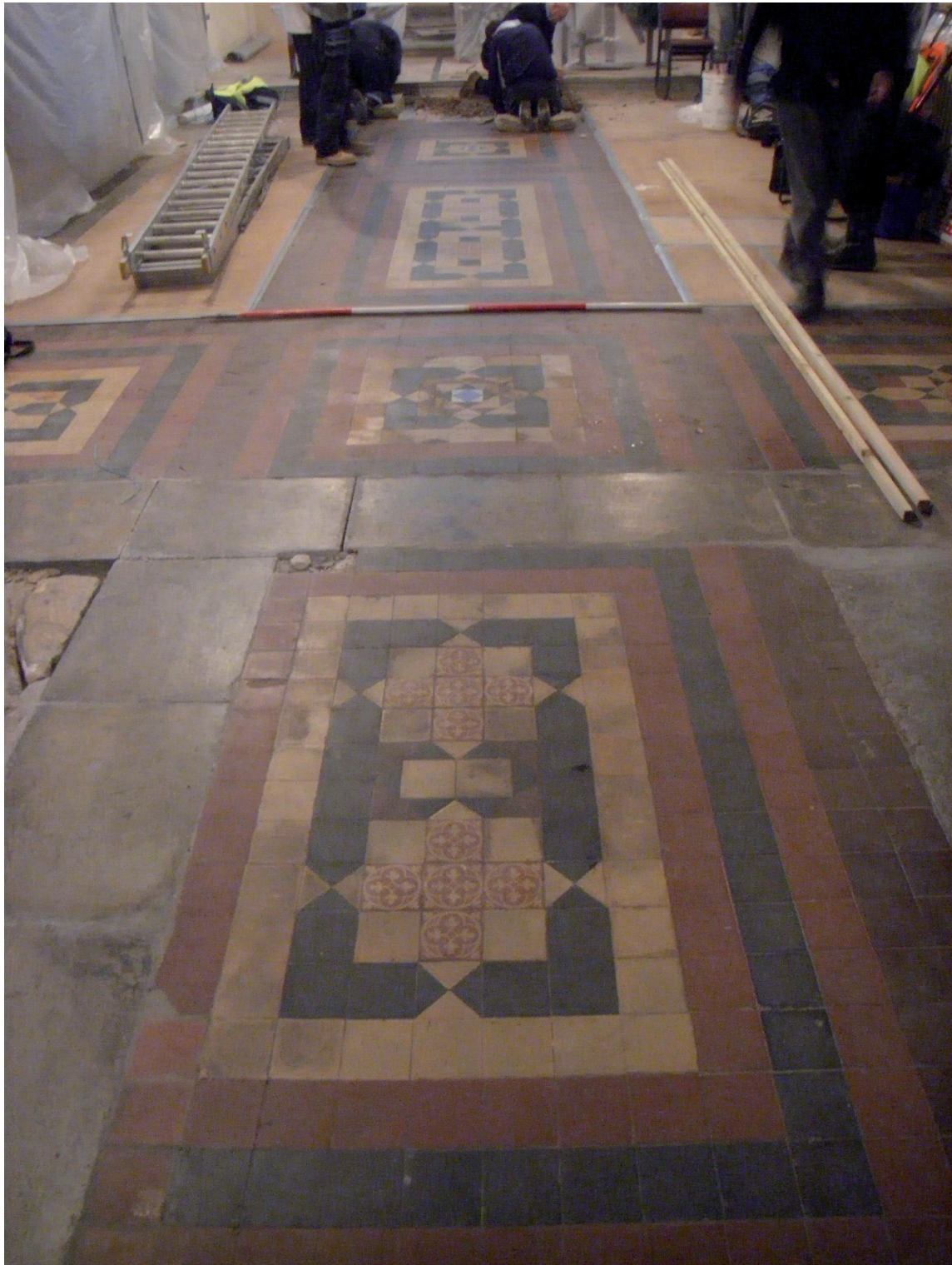
1. Trinity Chapel: Tiling prior to removal
