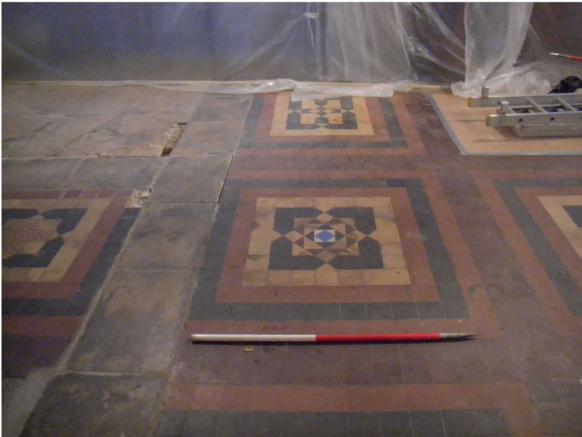
3. Trinity Chapel: Tiling prior to removal
