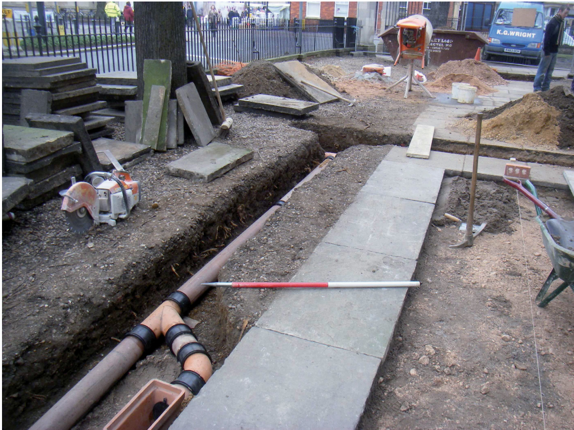
8. West End: Excavated drain trenches
