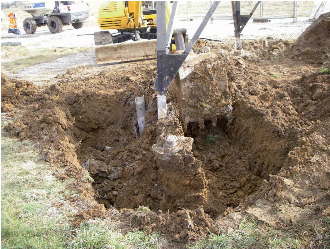
Figure 2: Pylon 147. Machine excavation of foundation pit
