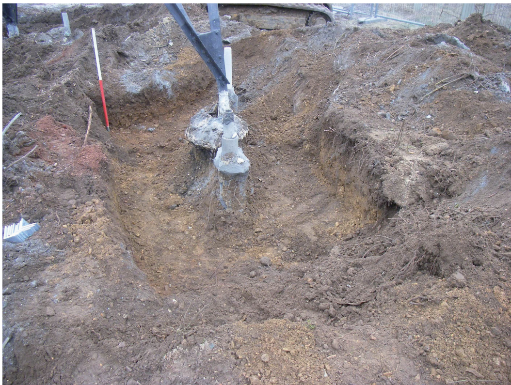
Figure 3: Pylon 145. Excavated foundation pit showing piles and existing pylon leg
