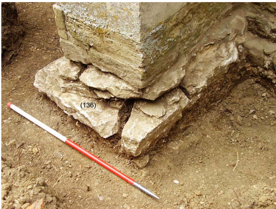
Plate 6: Buttress 3 padstones (136). Scale 1m
