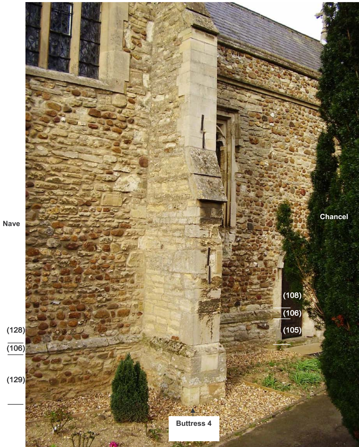
Plate 10: Nave, Buttress 4 and chancel. (post-reinstatement)
