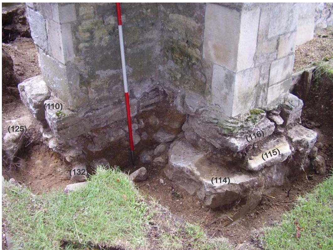
Plate 2: Chancel south-east corner double buttress. Scale 1m
