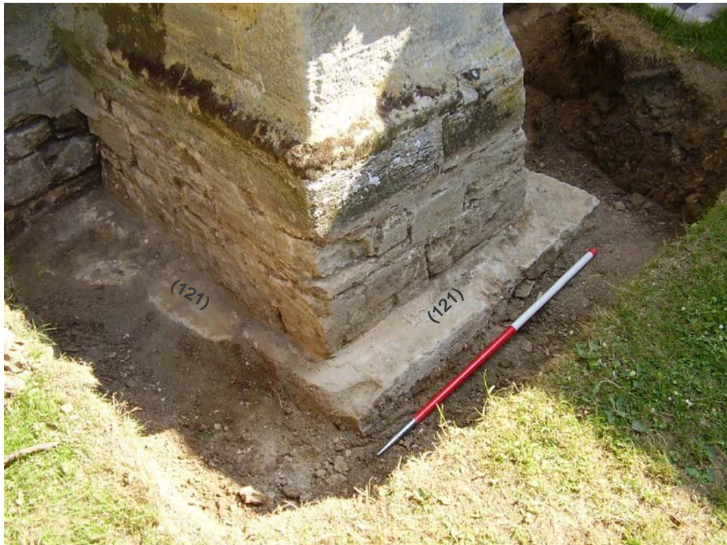
Plate 9: Tower padstones beneath Buttress 2. Scale 1m
