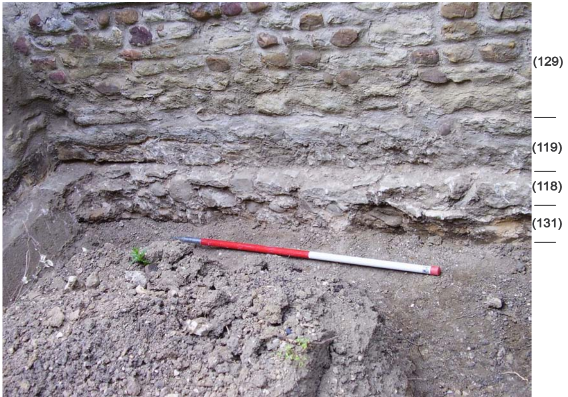
Plate 5: Nave foundation course (131), and plinth (118). Scale 1m
