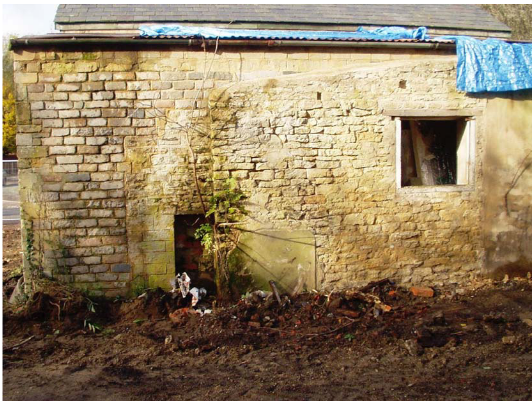
Photograph 1 Eastern elevation of shed, showing incorporation of earlier limestone outbuilding.
