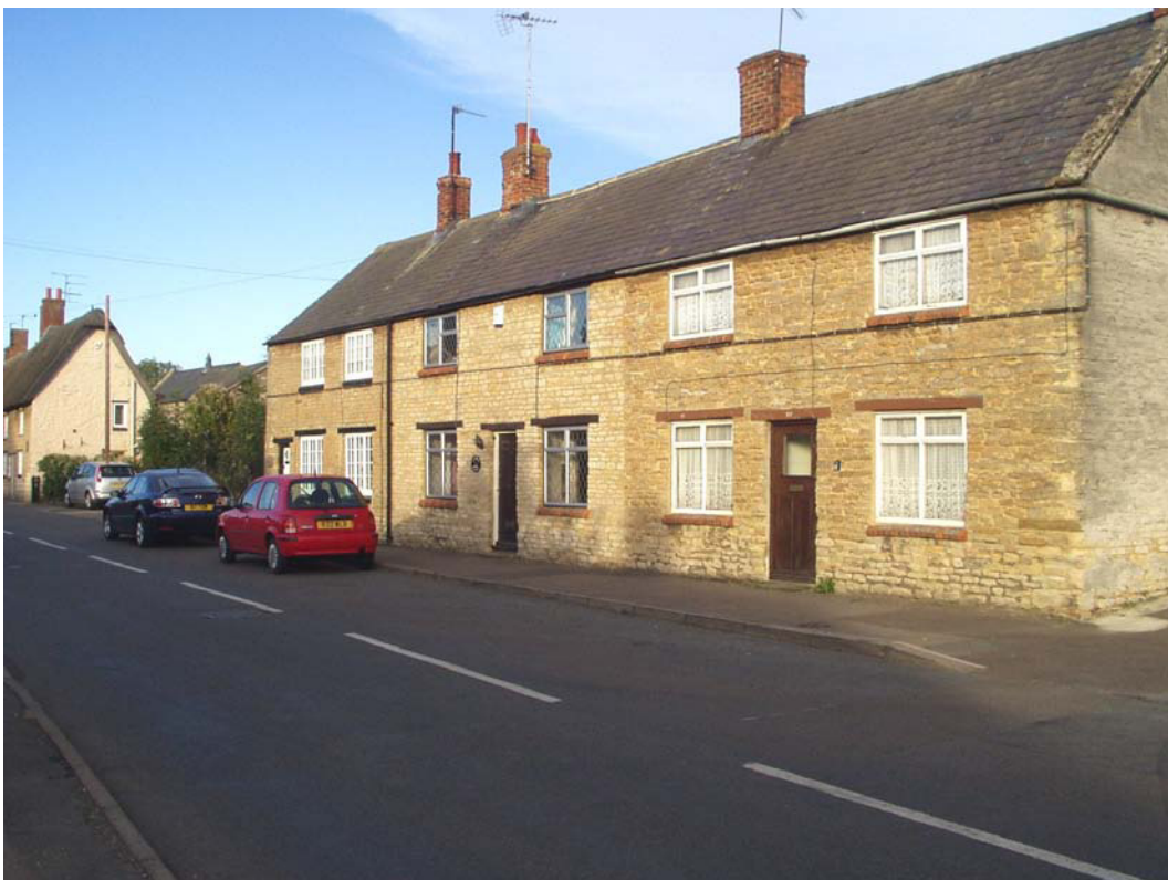
General view of remaining cottages immediately prior to site clearance in 2004. The gable end of the building at the left side of the image corresponds to the taller gable in the upper image.
