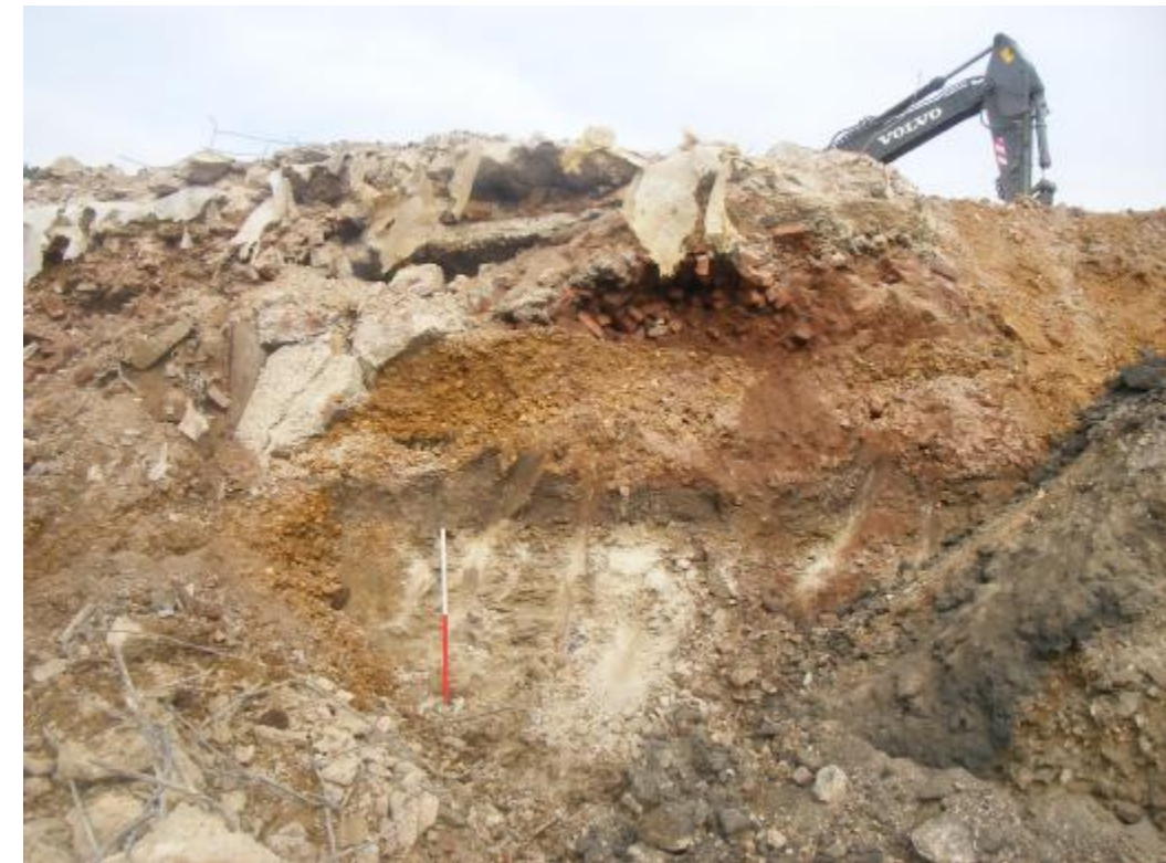
Plate 2: Zone 3, preserved subsoil and limestone deposits after removal of retaining wall facing north-east. 1m scale
