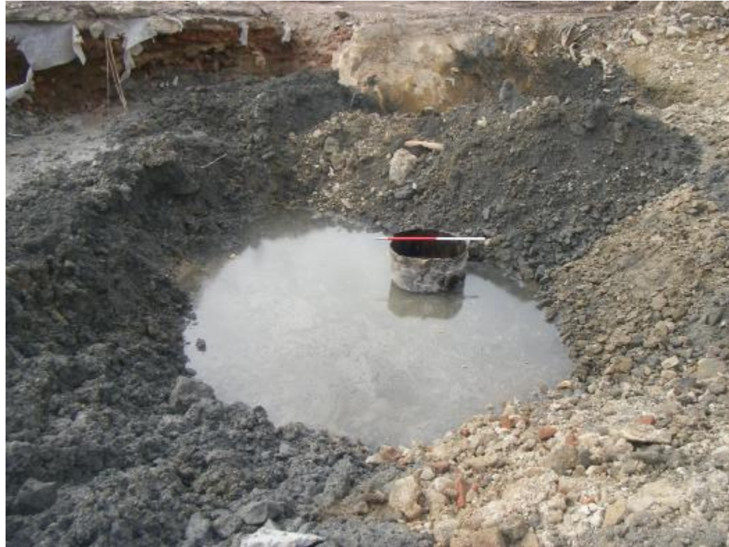
Plate 5: Zone 3 facing north-west showing exposed sump. 1m scale
