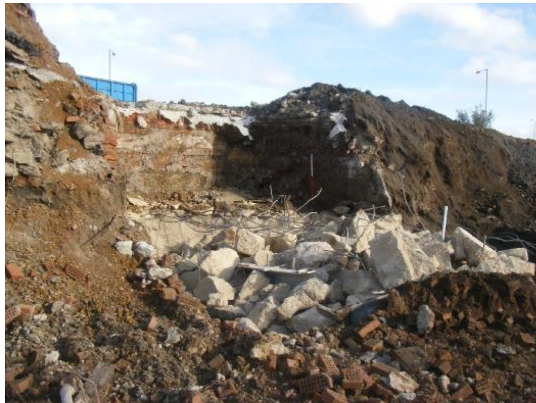
Plate 7: Zone 3 facing east showing scale of foundation slab. 1m scale
