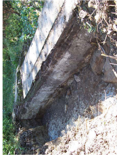
Trench 2 and weir retaining wall (205), looking south-east.
