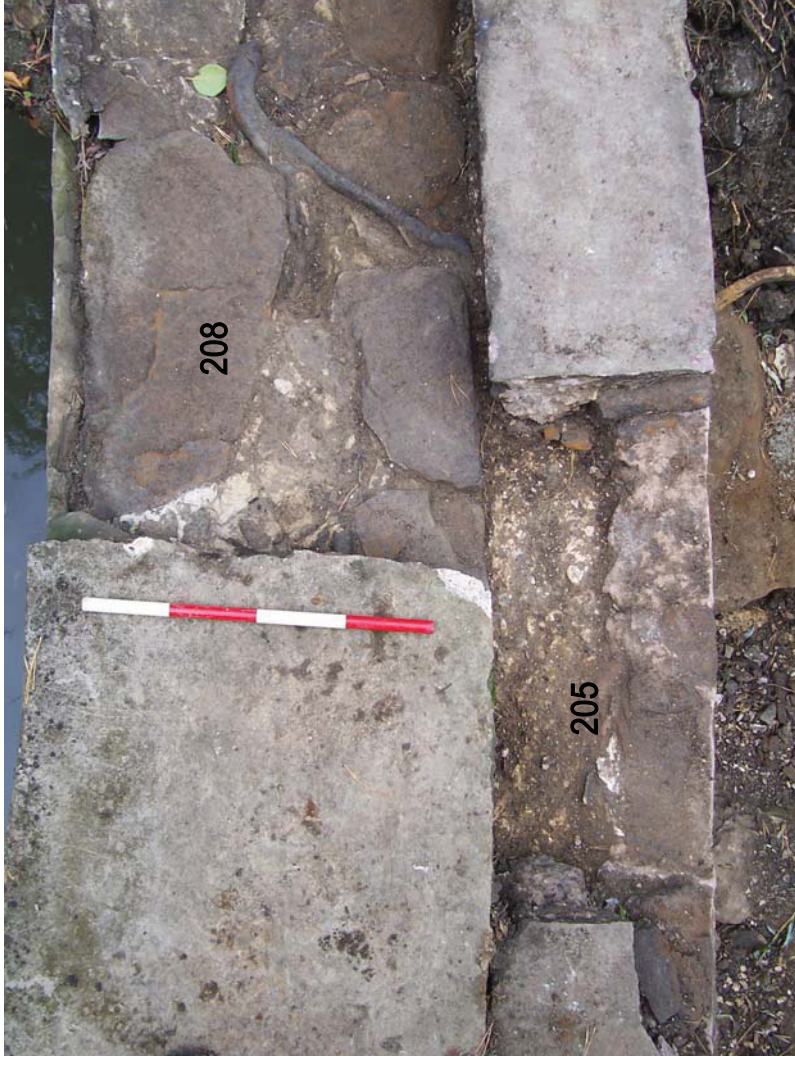
Top of weir wall (208) (top of picture) and 20 th century retaining wall (205) (bottom of picture), after removal of sections of the concrete capping. Scale 40cm
