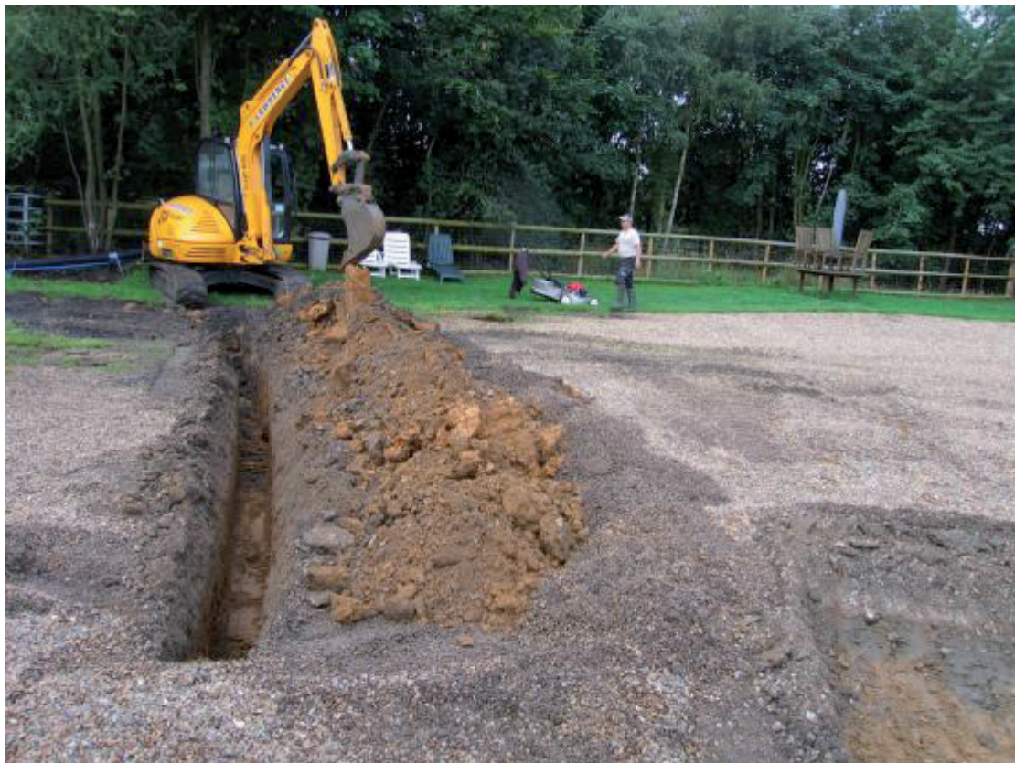
Water pipe trench, looking south
