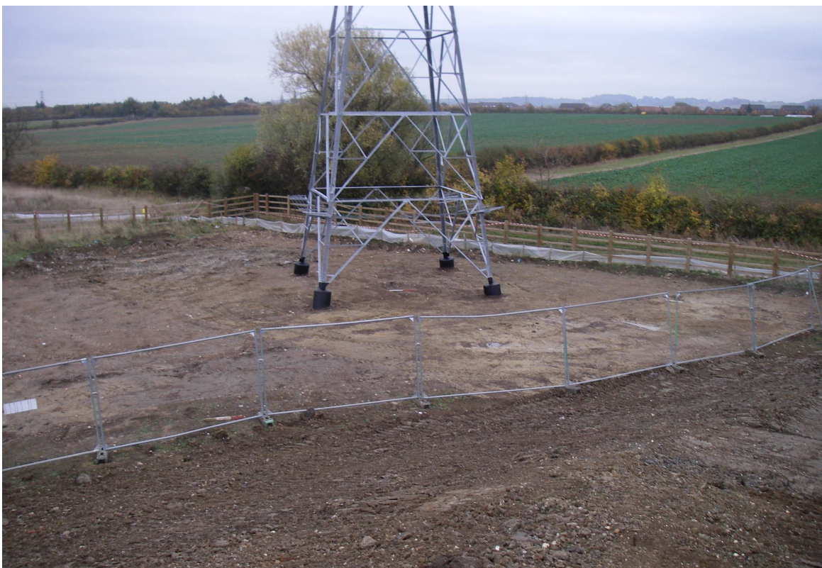
Figure 4: Pylon 110. Re-stripped piling mat area following construction of pylon
