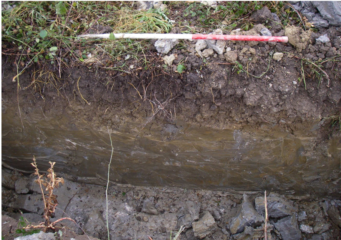
Figure 3: Pylon 110. Trench for removal of old foundation
