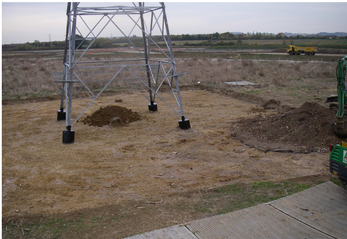
Figure 6: Pylon 111. Re-stripping of piling mat area following construction of pylon
