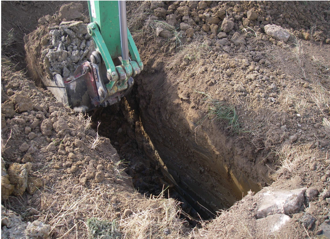
Figure 5: Pylon 111. Trench for removal of old foundation
