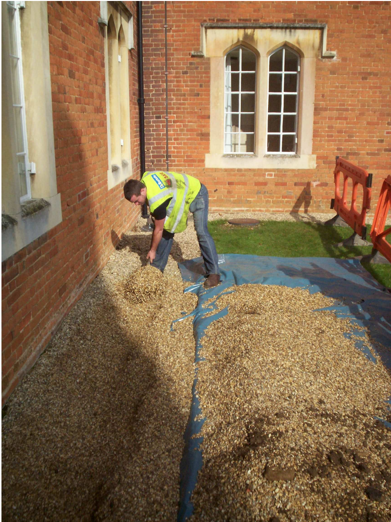
Figure 2: Removal of French drain gravel fill prior to installation of cable
