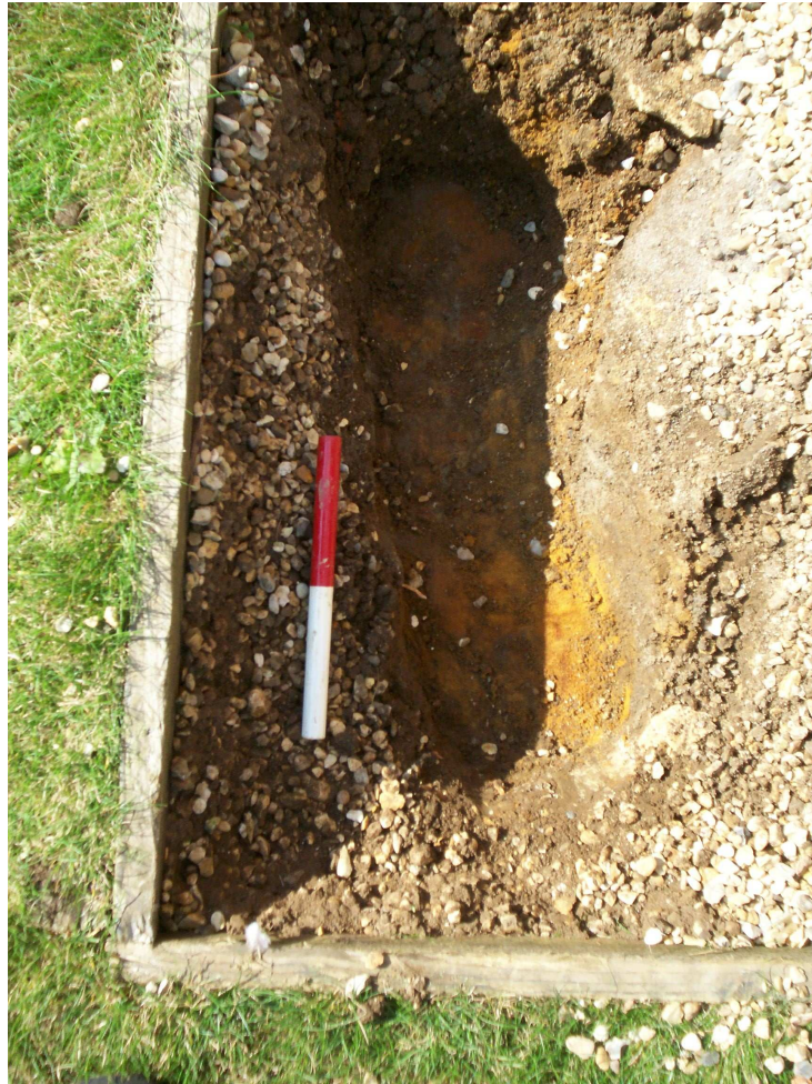
Figure 4: Exposure of sandstone within turning chamber excavation
