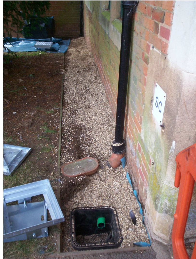
Figure 3: Installation of turning chamber
