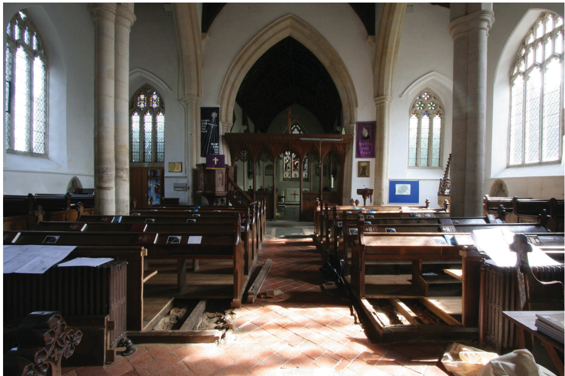
Figure 4: Location of works in nave
