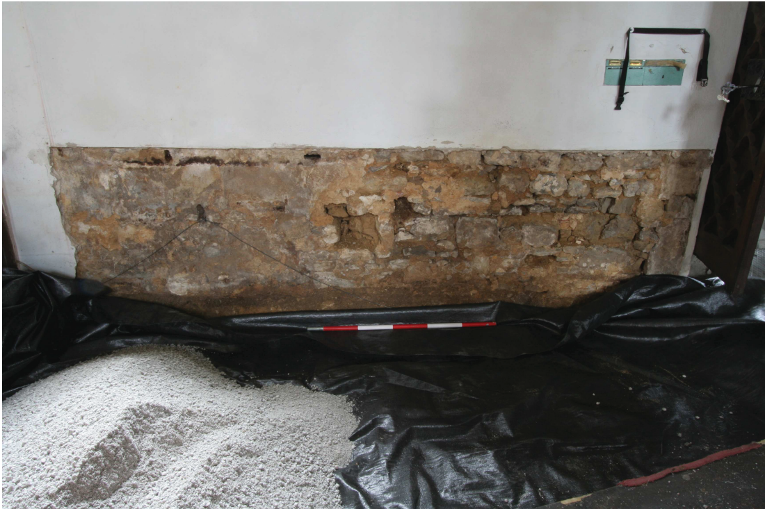
Figure 5: Exposed masonry in north aisle
