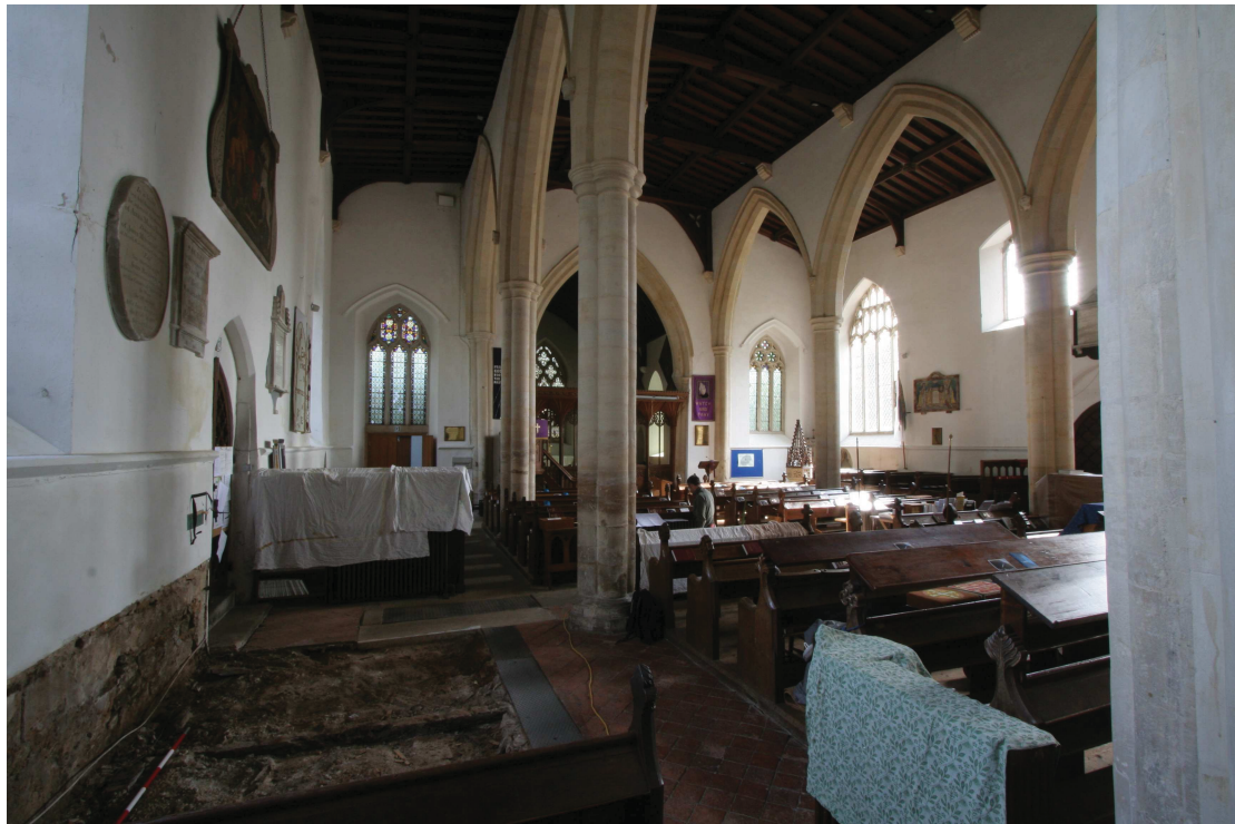
Figure 3: Location of works in north aisle
