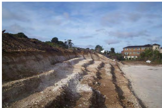
East end of Area 3, looking west
