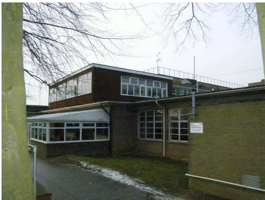
Plate 15: Single Storey Block at End of North-Eastern Wing
