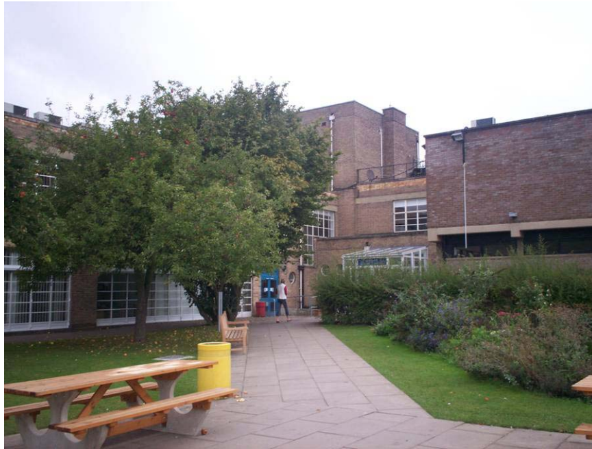
Plate 13: South Western and North-Eastern Wings from Courtyard
