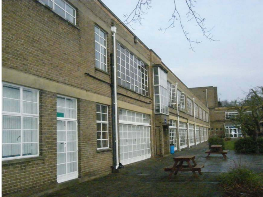
Plate 9: South-East Elevation of South-Western Arm
