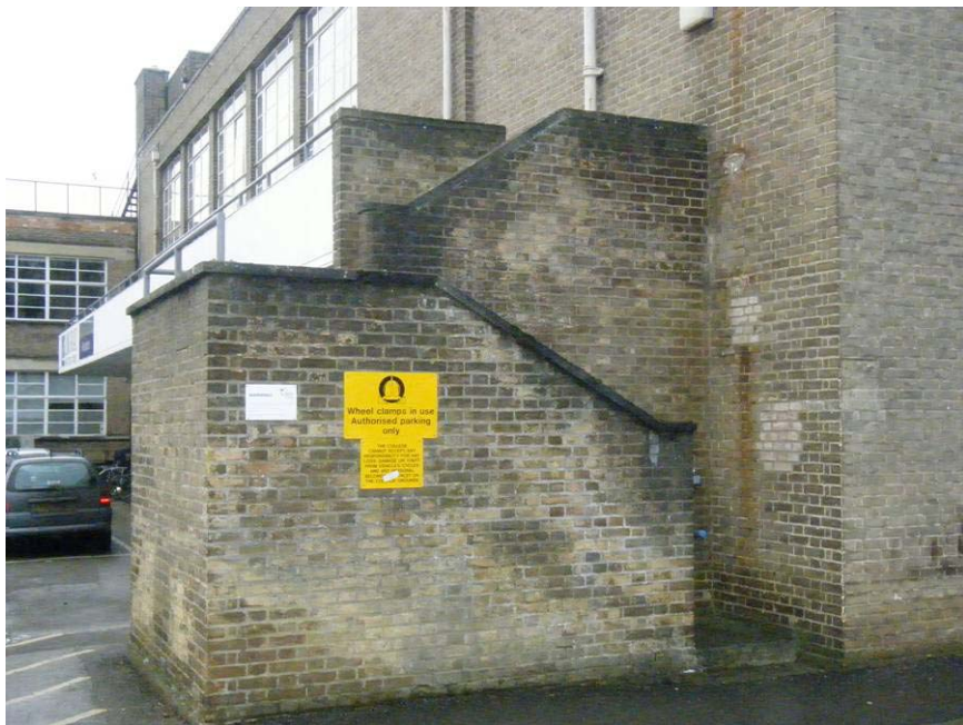
Plate 18: Details of Stairs up to First Floor Balcony
