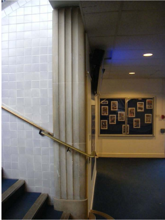
Plate 19: Internal Detail Main Stair Case
