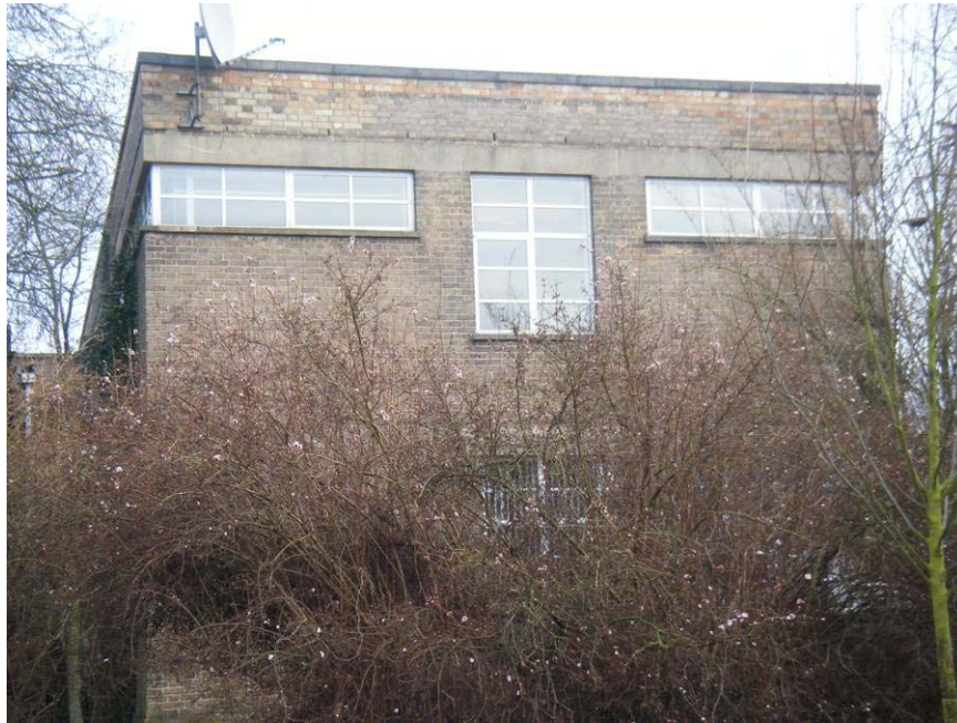
Plate 7: South-West End of South-Western Block (Former Library Windows)
