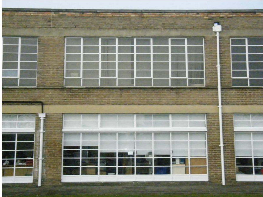
Plate 11: Detail of Windows, South-East Elevation, South-Western Wing
