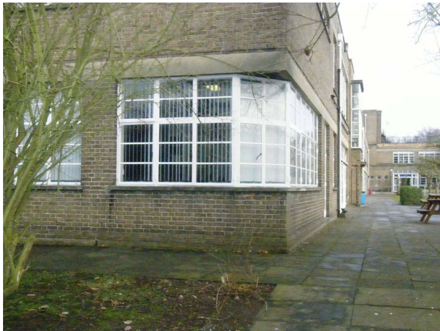
Plate 8: Detail of Window, South-West End of South-Western Block (Former Geography Room)
