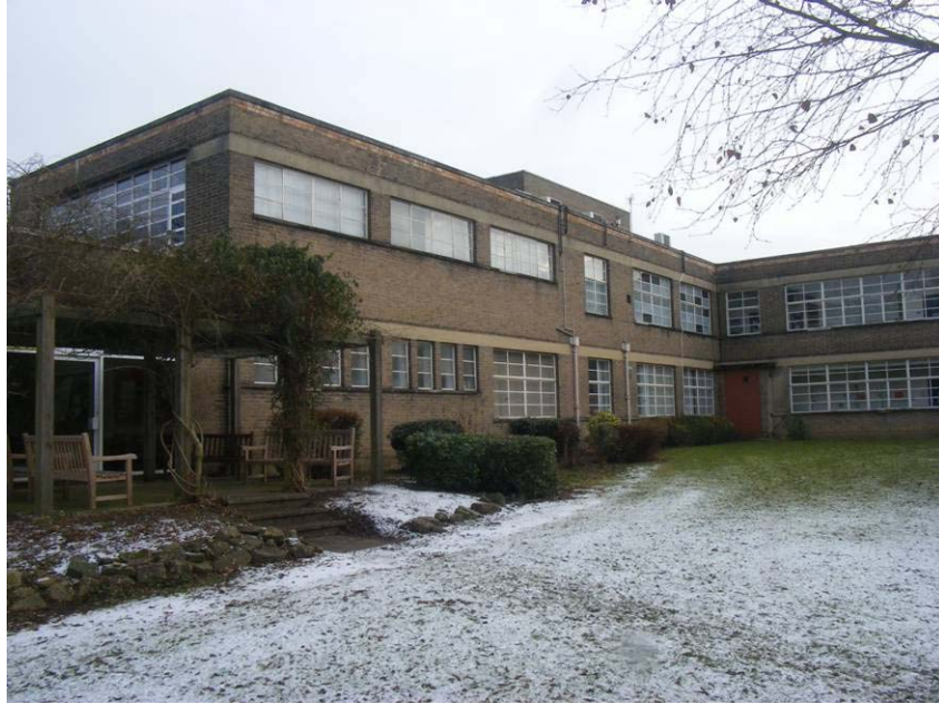
Plate 5: North-Western Block, Former First-Floor Art Room and Ground-Floor Administration
