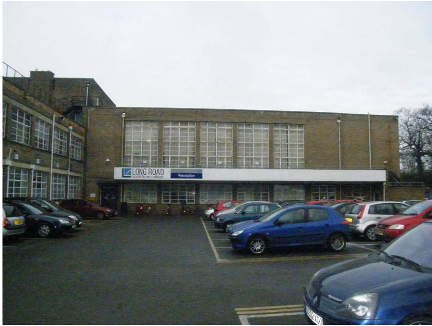
Plate 17: North-Eastern Wing: Main Hall
