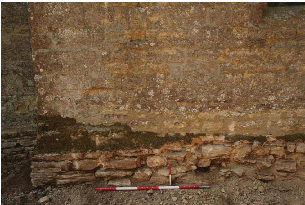
Figure 16: Nave north-east corner. 1m and 0.20m scales
