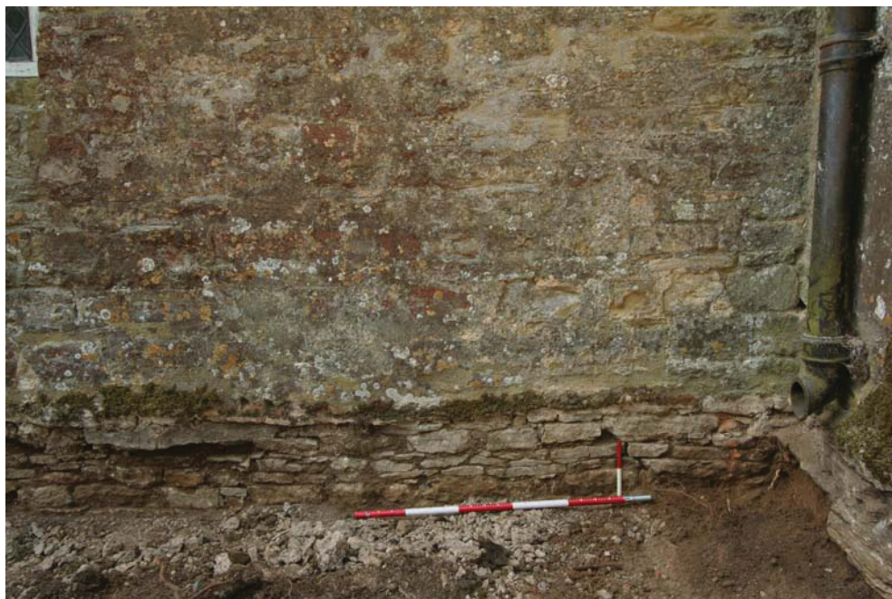
Figure 14: Chancel north-west corner. 1m and 0.20m scales
