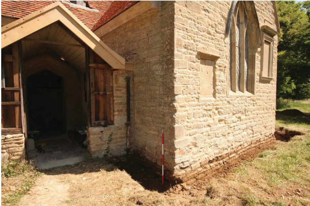
Figure 3: Porch and transept. 1m scale
