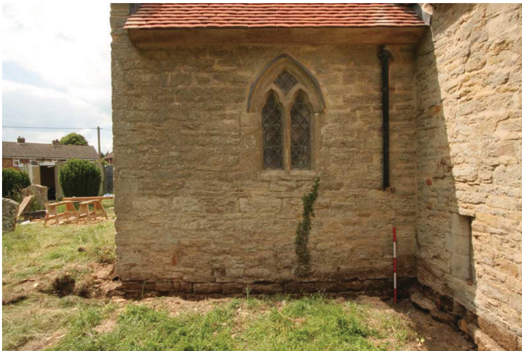
Figure 4: Transept east wall. 1m scale
