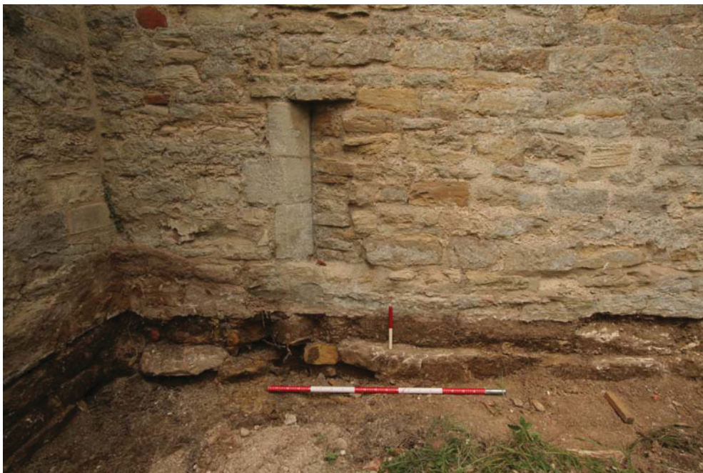
Figure 6: Transept and chancel south corner. 1m and 0.20m scales
