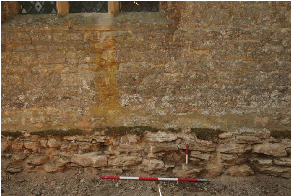
Figure 17: Nave north wall central east area. 1m and 0.20m scales
