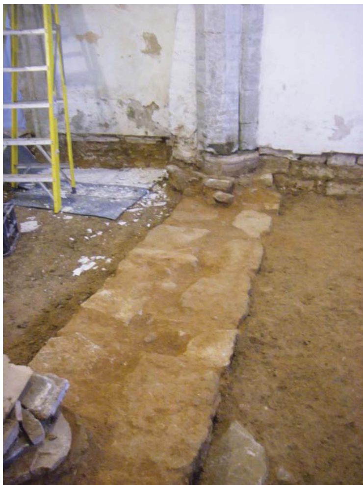
Figure 25: Exposed wall foundation looking east
