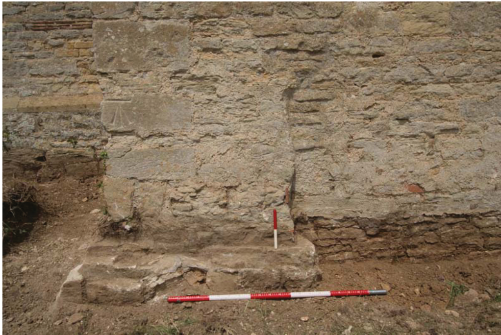
Figure 21: Nave south-west corner buttress. 1m and 0.20m scales
