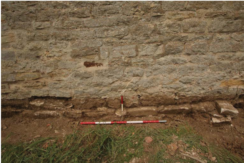
Figure 7: chancel south wall central area. 1m and 0.20m scales
