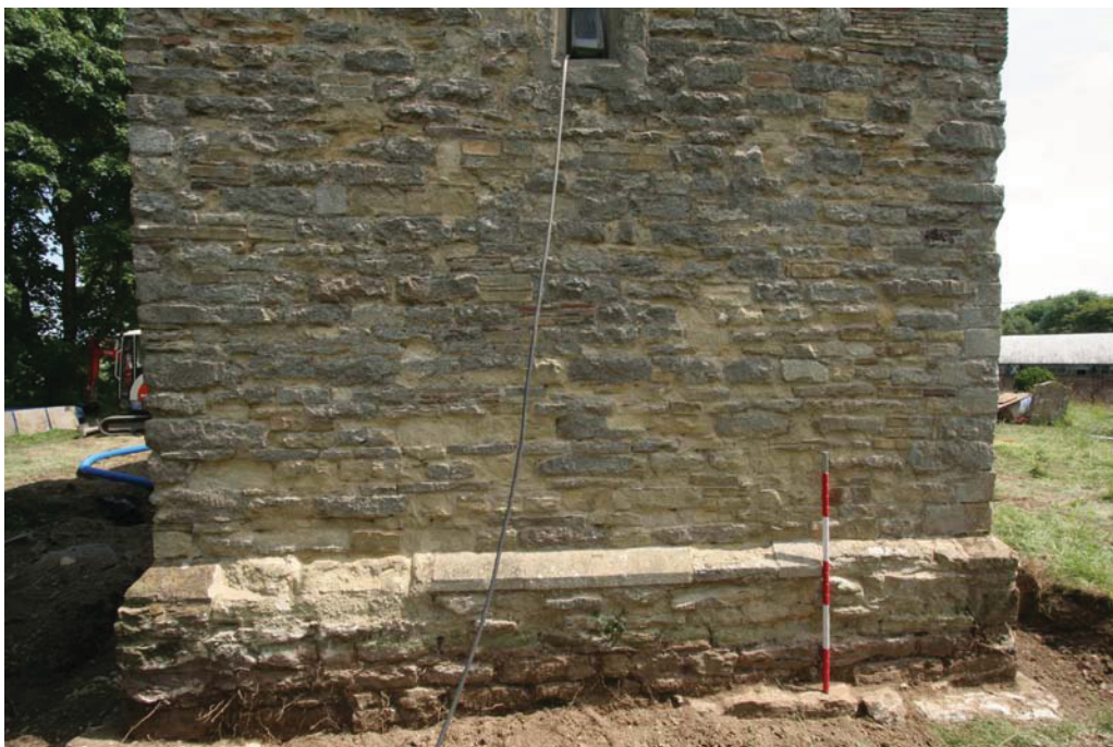
Figure 20: Tower west wall. 1m scale
