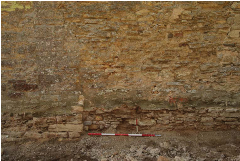
Figure 18: Nave north wall central west area. 1m and 0.20m scales
