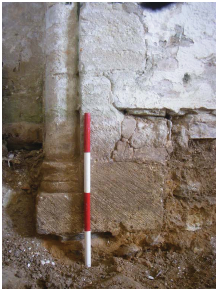
Figure 29: Exposed chancel arch respond footing. 0.40m scale
