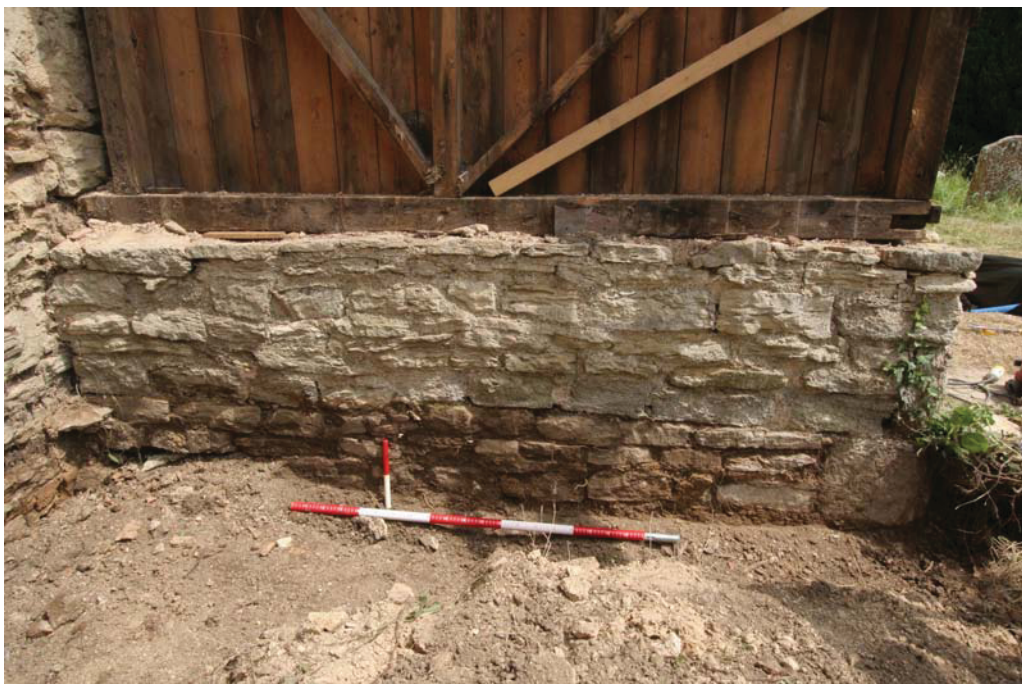
Figure 22: Porch west wall. 1m and 0.20m scales
