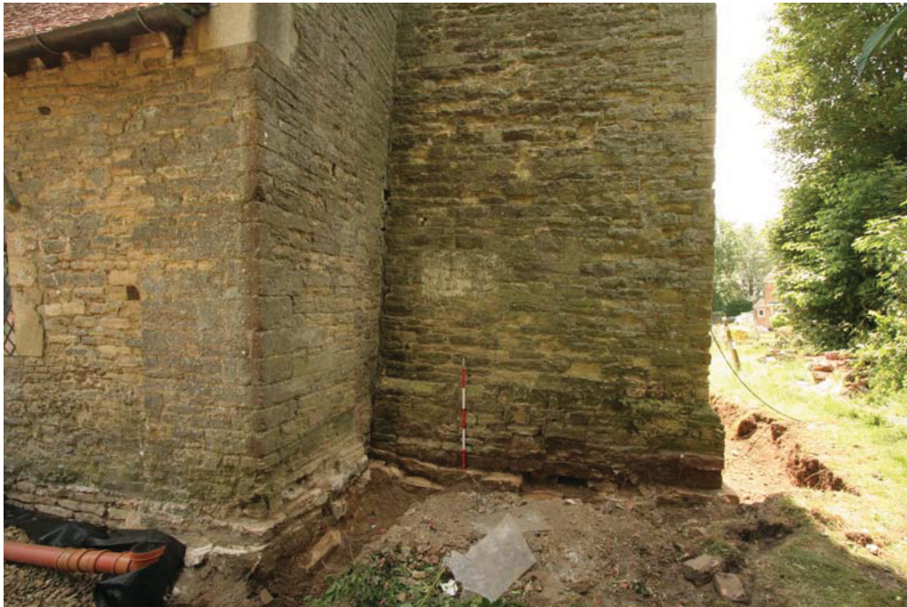
Figure 19: Nave and tower north-west corner. 1m scale
