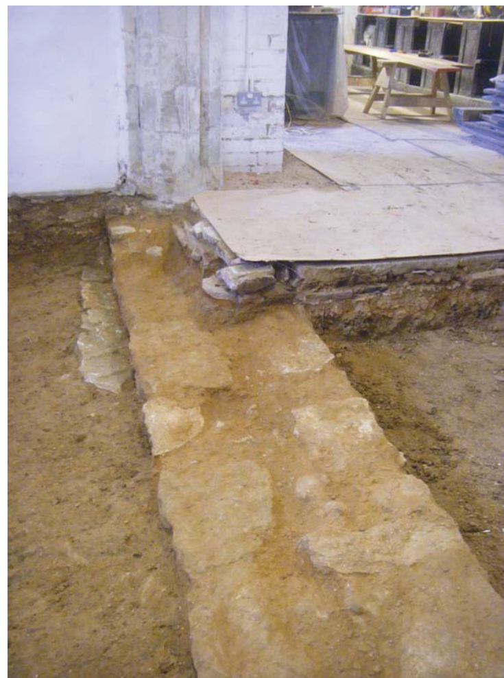
Figure 26: Exposed wall foundation looking west
