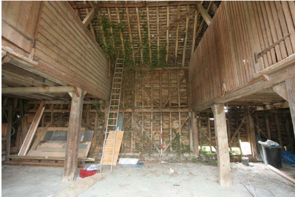
Plate 5: Interior view of central bay looking north
