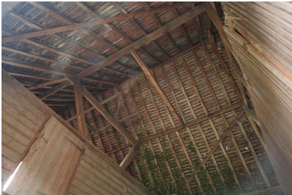
Plate 6: Interior view of roof structure
