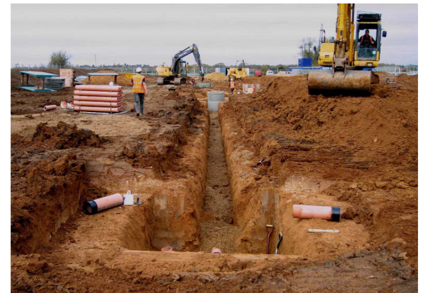
Photograph 2: machining of trench for storm drain
