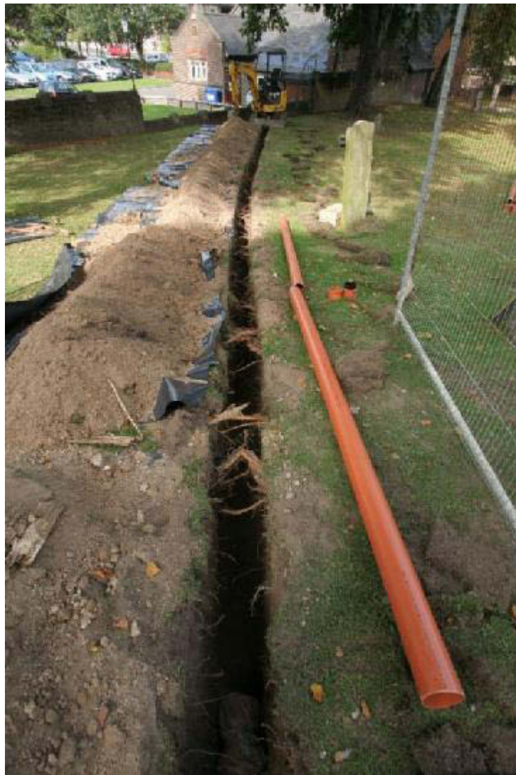
Figure 10: Foul water drain looking north-west towards Church Hall
