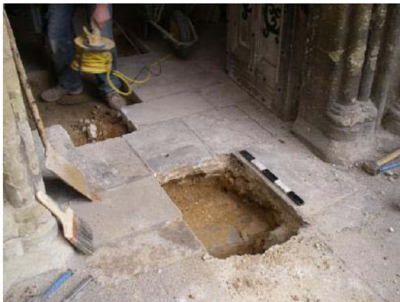
Figure 11: Dressed foundation or threshold blocks within north-west doorway
