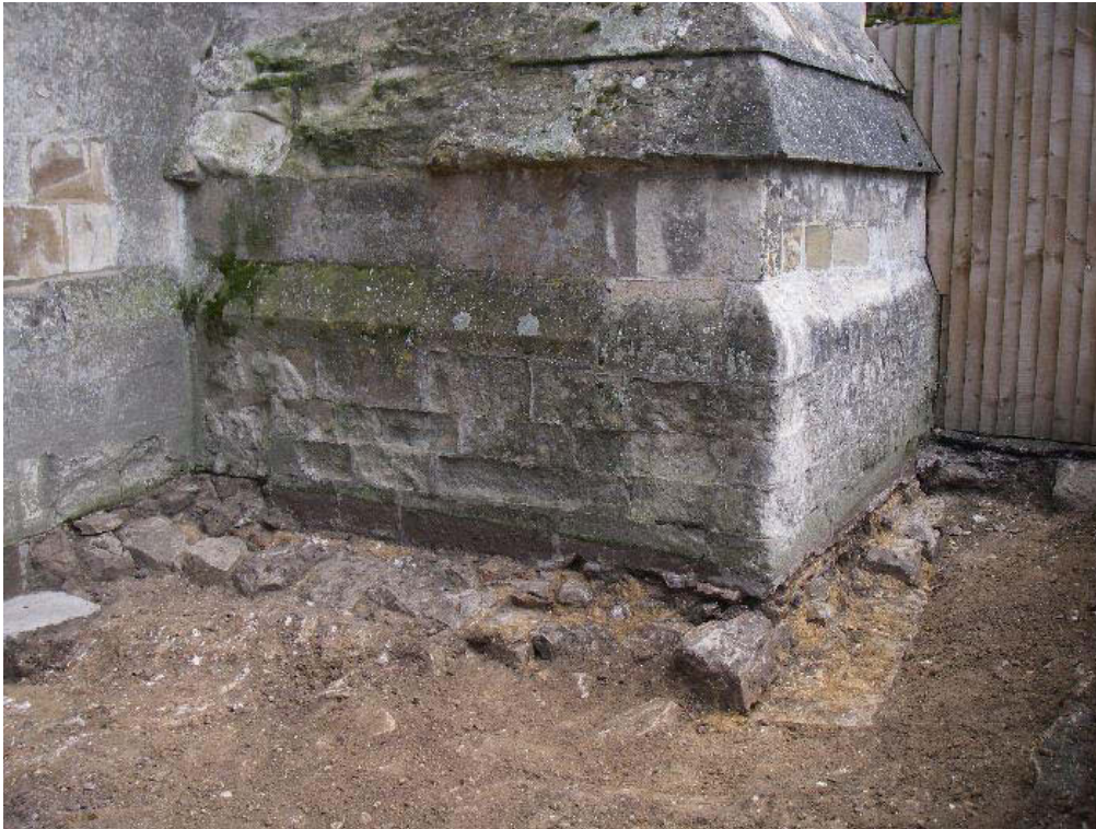
Figure 7: Foundation of south-western buttress in plan
