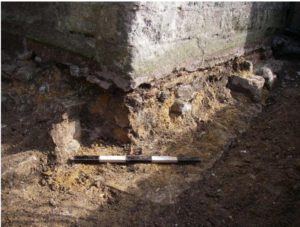
Figure 8: Foundation of south-western buttress elevation detail
