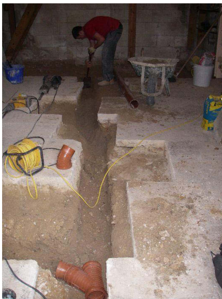
Figure 12: Foul water drain inside entrance lobby (fully excavated)
