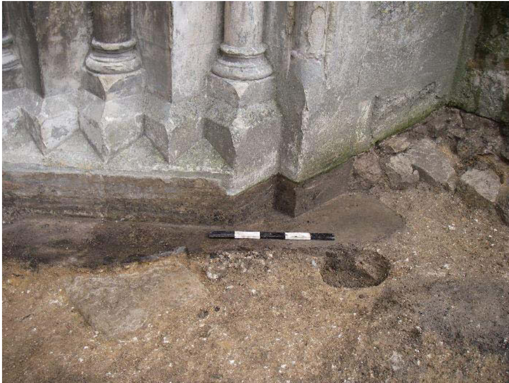
Figure 5: Early 20th-century paving slabs and make-up layers (0.5m scale)
