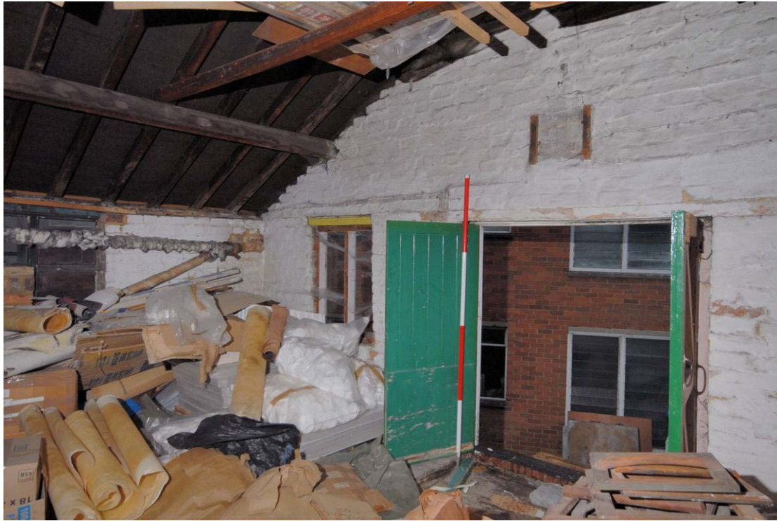
Plate 21: First floor workshop H
