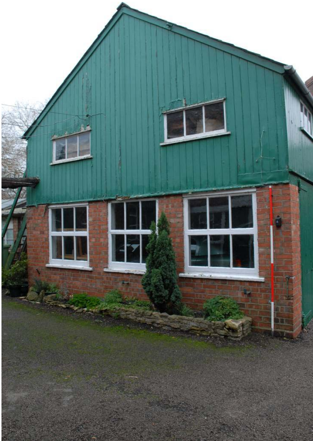
Plate 6: NW elevation (garage L)
