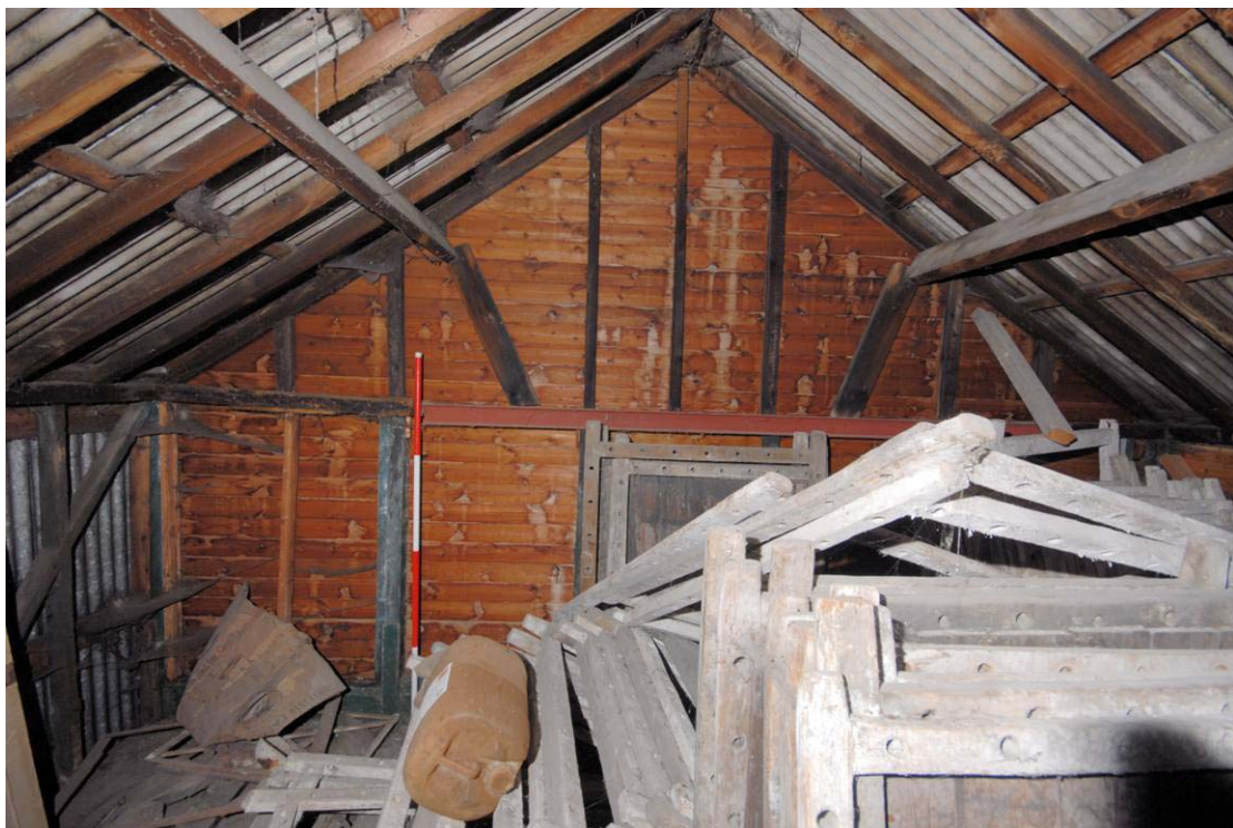
Plate 24: First floor above area J (southern end of building)
