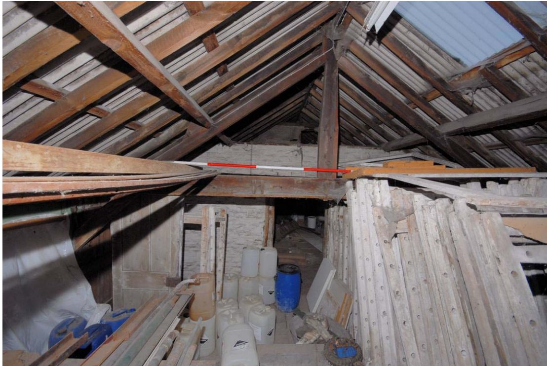
Plate 23: First floor above area E/F, view towards area D
