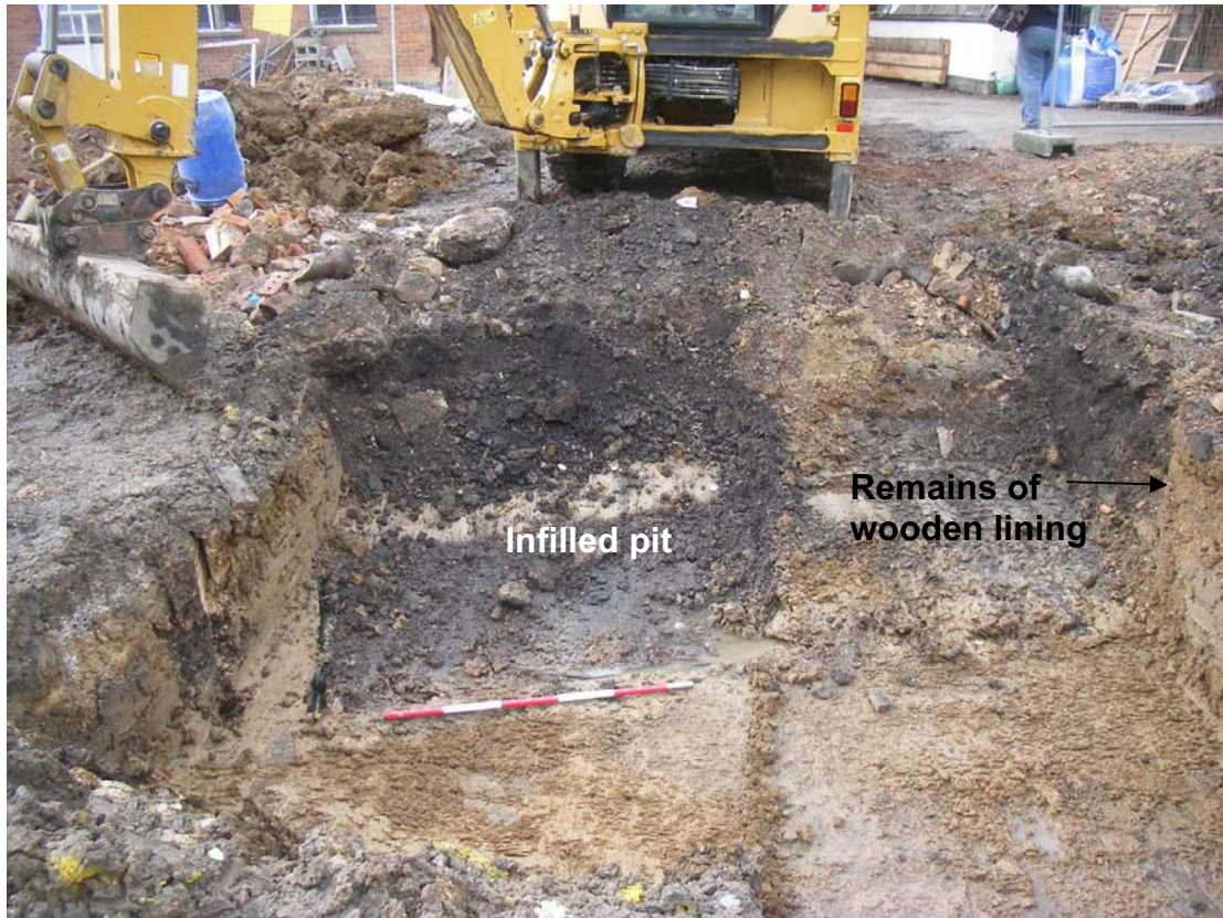
Plate 34: Infilled soaking pit in Test Pit 1 (former wet yard area A. Photograph taken by Mark Phillips)
