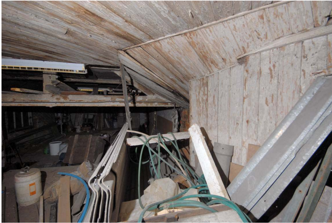
Plate 25: First floor above area C, view towards area D
