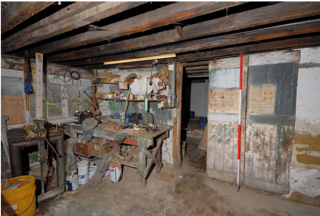
Plate 16: Workshop area D, view towards drying area F
