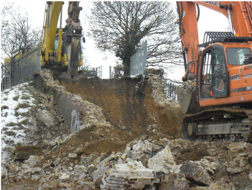
Figure 9: Dog Kennel Bridge demolished. Southern abutment. (Photo: Albion Archaeology)
