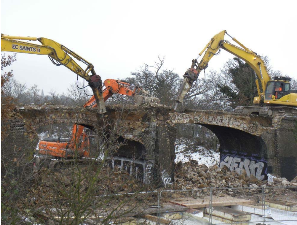
Figure 8: Dog Kennel Bridge under demolition. West facing elevation. (Photo: Albion Archaeology).
