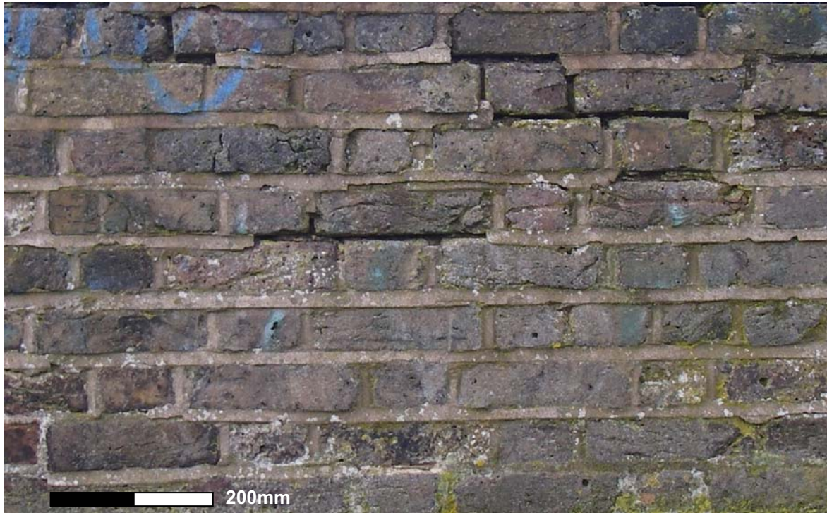
Figure 10: Western bridge parapet, internal view, brick detail. Change from old Flemish coursing (left) to English coursing of extension (right). (Photo: Albion Archaeology)
