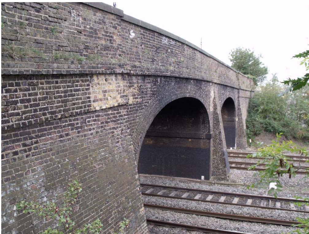
Figure 7: Dog Kennel Bridge east facing elevation. Southern Brunel arch with sooting in foreground of photograph. (Photo: Albion Archaeology)
