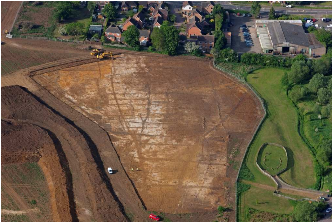
Earthmoving (nearing completion) exposes Roman ditches (dark linear soil marks) which divided the settlement up into a series of enclosures adjacent to a trackway (defined by two parallel ditches). The small yellow dots are archaeologists!
