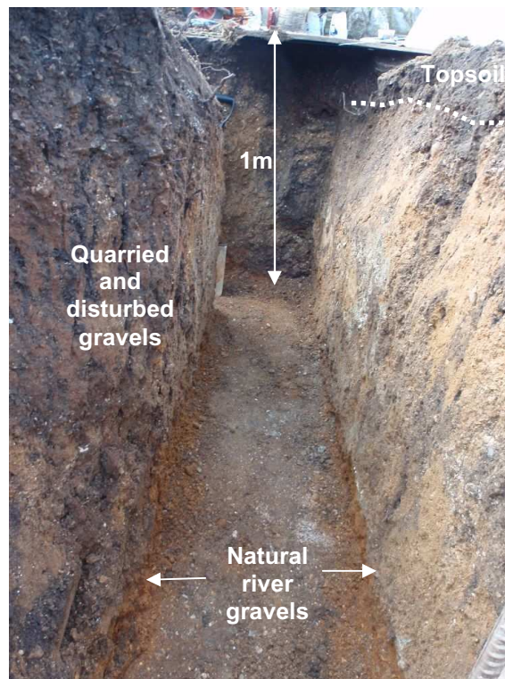
Figure 3: New extension — foundation trench looking north.
