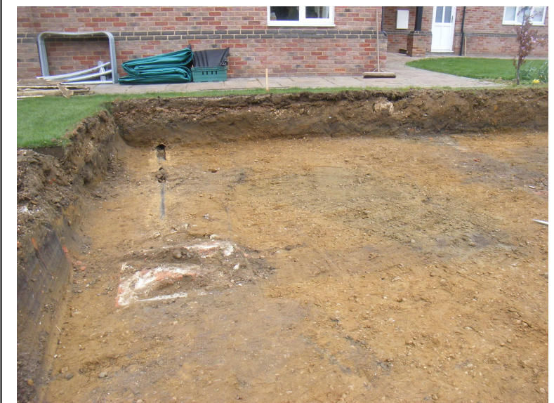
East half of PDA showing foundations and drains. Looking ENE.
