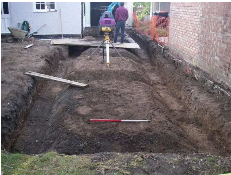
Figure 2c: Excavated foundation trenches, looking south, 1m scale.
