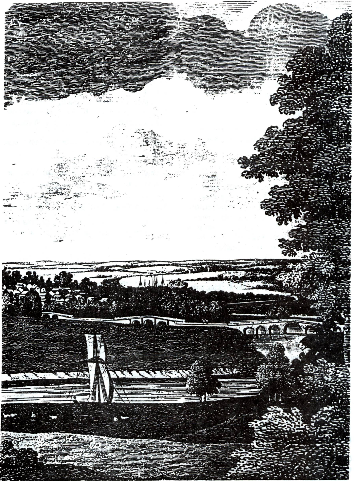
Figure 22: Pershore Bridge (HWCM 5574) - detail from an engraving by Thomas Sanders, 1779
