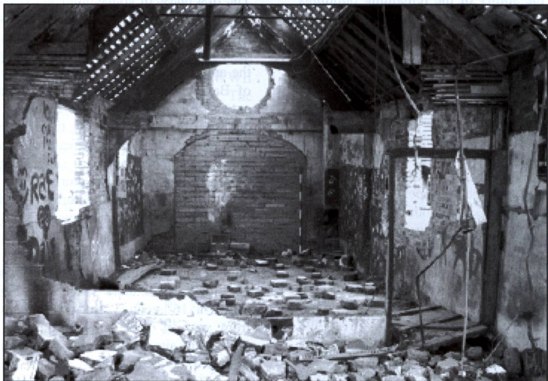
Fig. 44: Building 4 north and east elevations (above) and interior, looking east (below)
