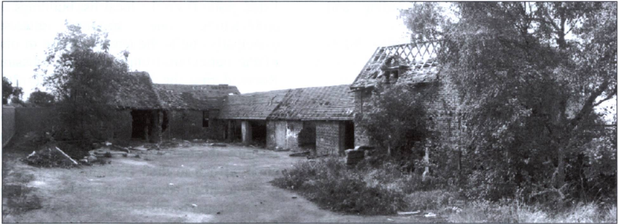
Fig. 41: Barn Farm, from entrance looking north
