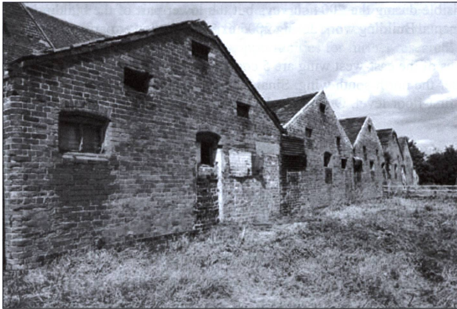
Fig. 8: South-facing elevation of the model farm
