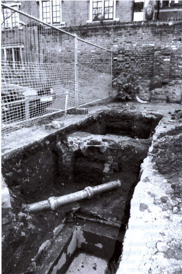
Fig. 66: Taylors Lane excavations, showing brick relieving arches in Trench 1
