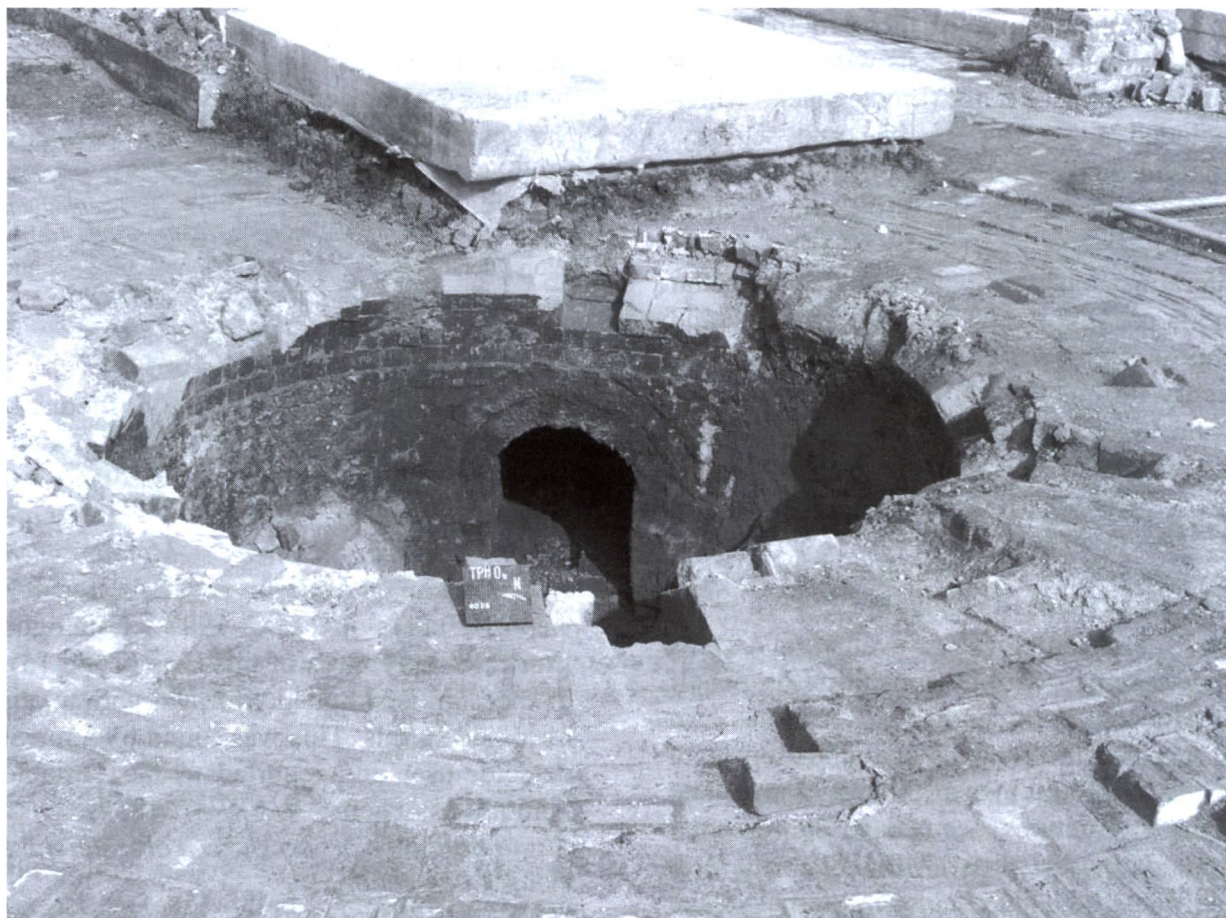
Fig. 21: Central well and exit flue of downdraught pottery oven, Trent Pottery, Stoke-on-Trent
