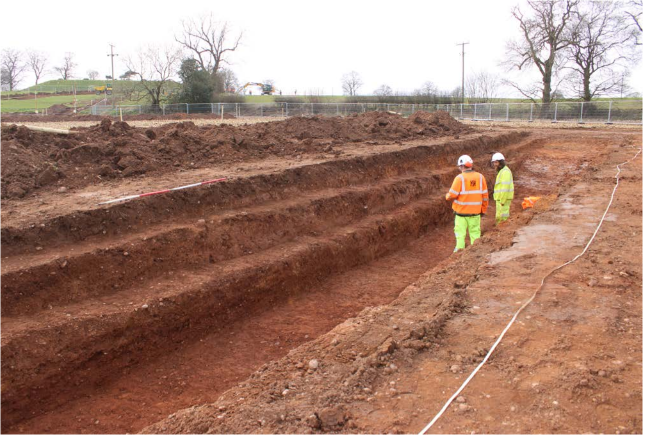
FIG 17 Working shot of Trench 13 after stepping
