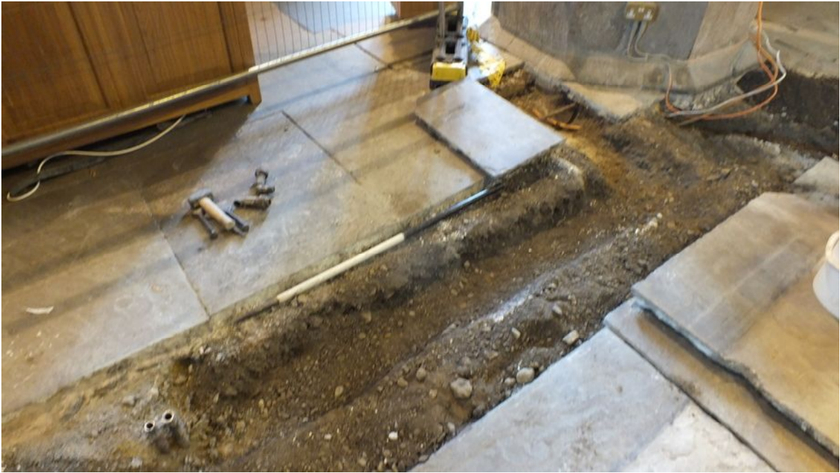
Plate 5: Trench C, viewed from the north-east
