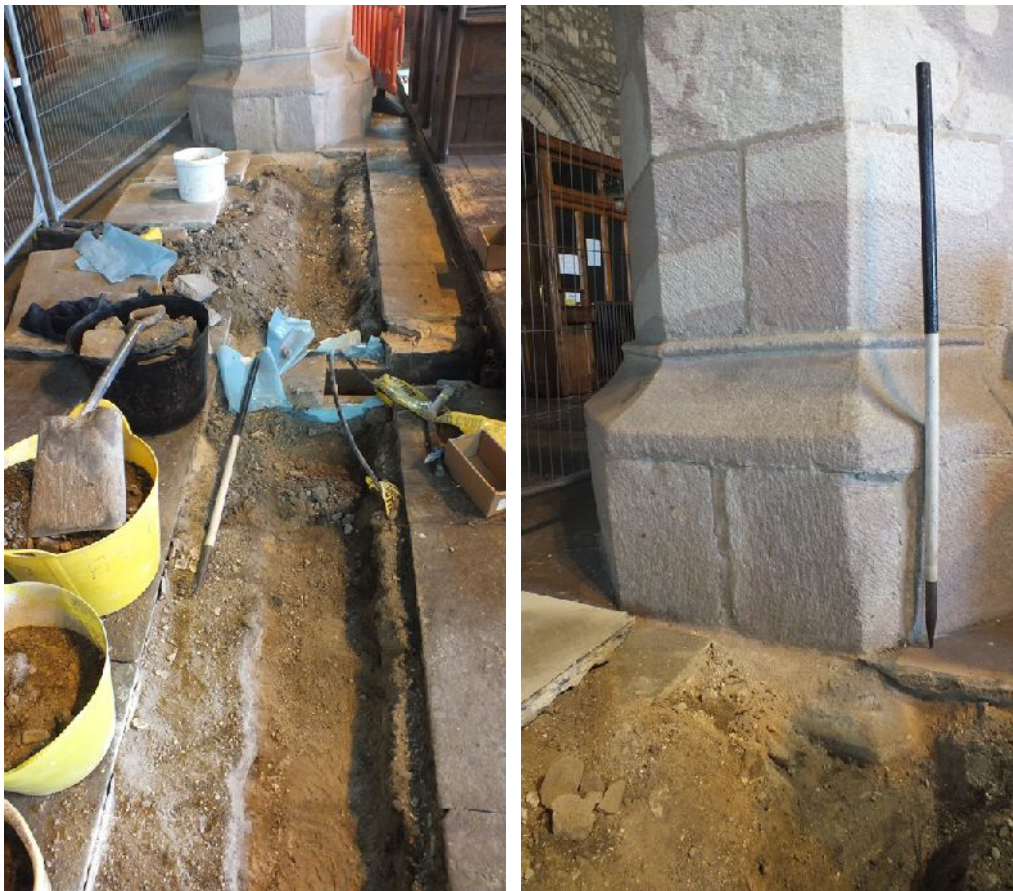
Plate 1 (left): Trench A excavated, viewed from the west
