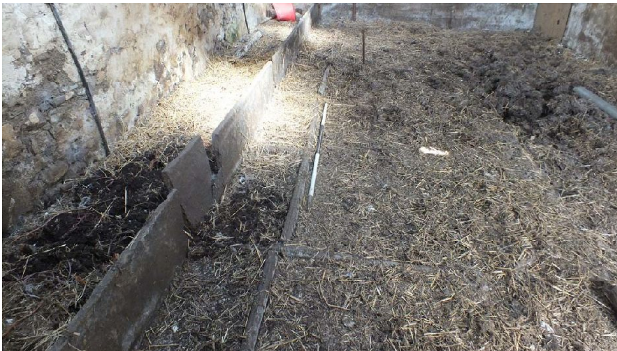
Plate 52: Stone divisions for troughs in Building C, from the south-east
