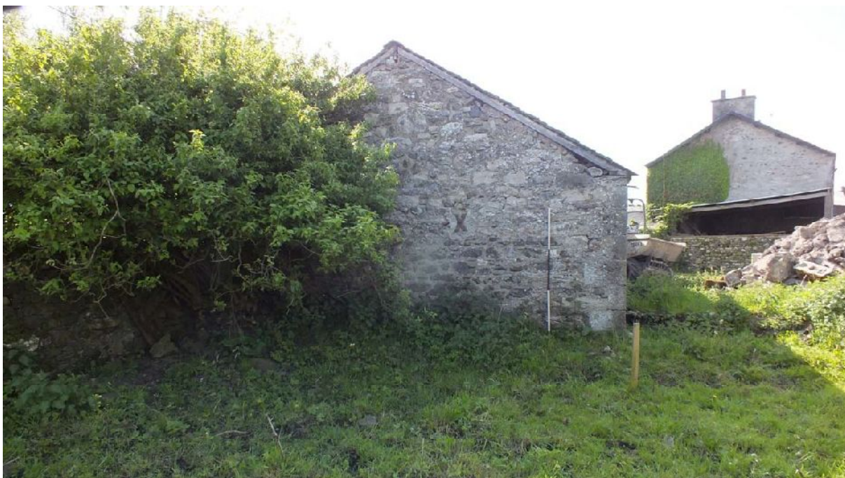
Plate 17: North-west external elevation of Building C, from the north-west
