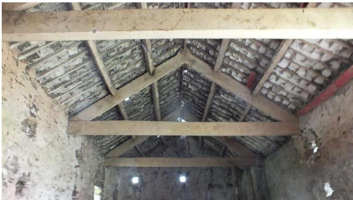
Plate 31: Trusses in upper floor of Building A, from the west
