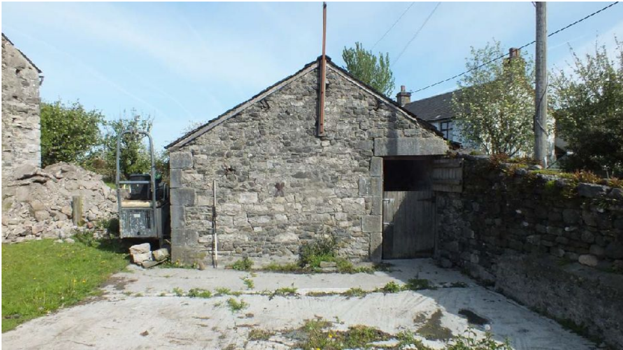
Plate 19: South-east external elevation of Building C, from the south
