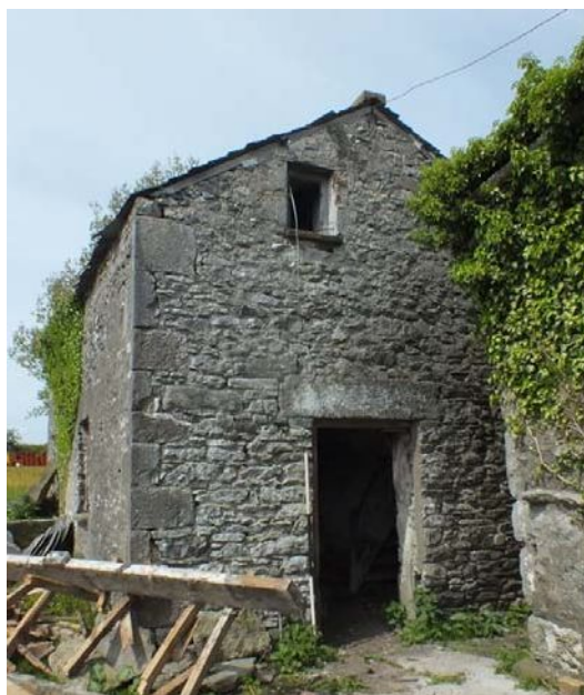
Plate 16 (left): East elevation of Building B, from the east
