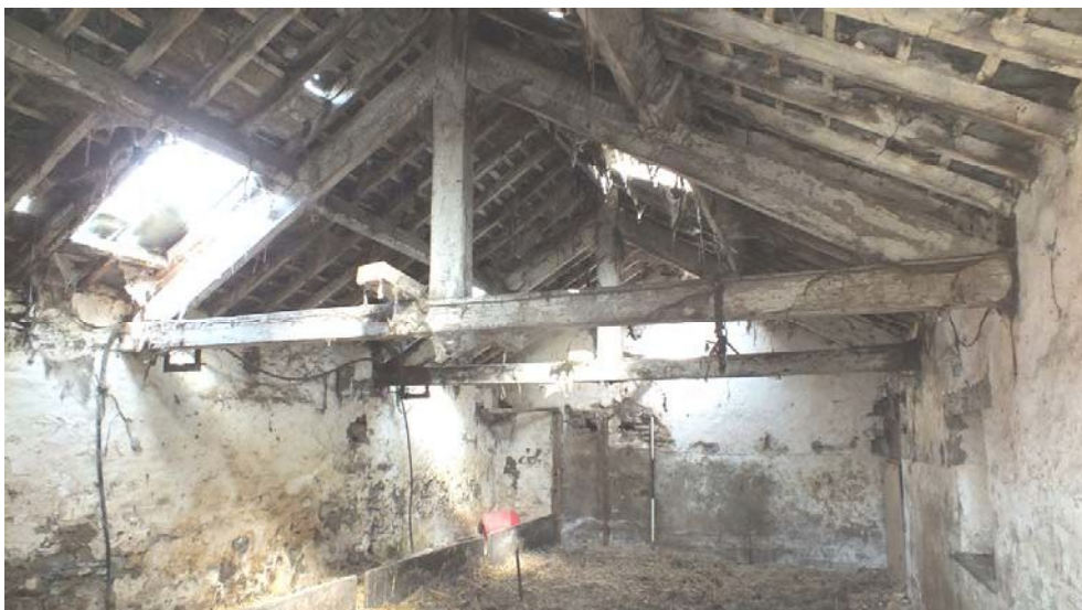
Plate 53: Trusses in Building C, from the south-east
