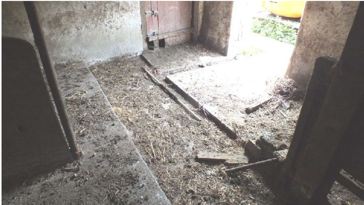
Plate 23: Dung channel in floor in lower floor Building A, lower floor Room 2, from the north-west
