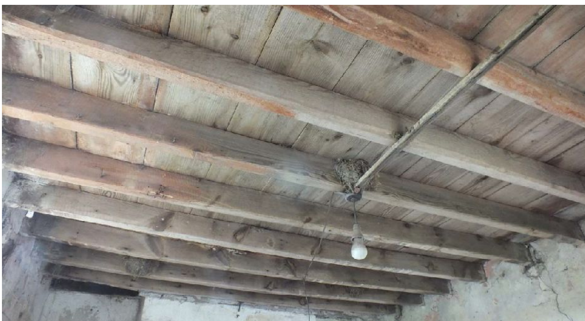
Plate 38: Ceiling in lower floor Room 1 of Building B, from the east
