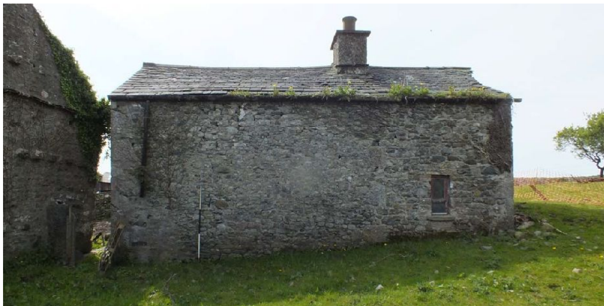
Plate 13: North elevation of Building B, from the north
