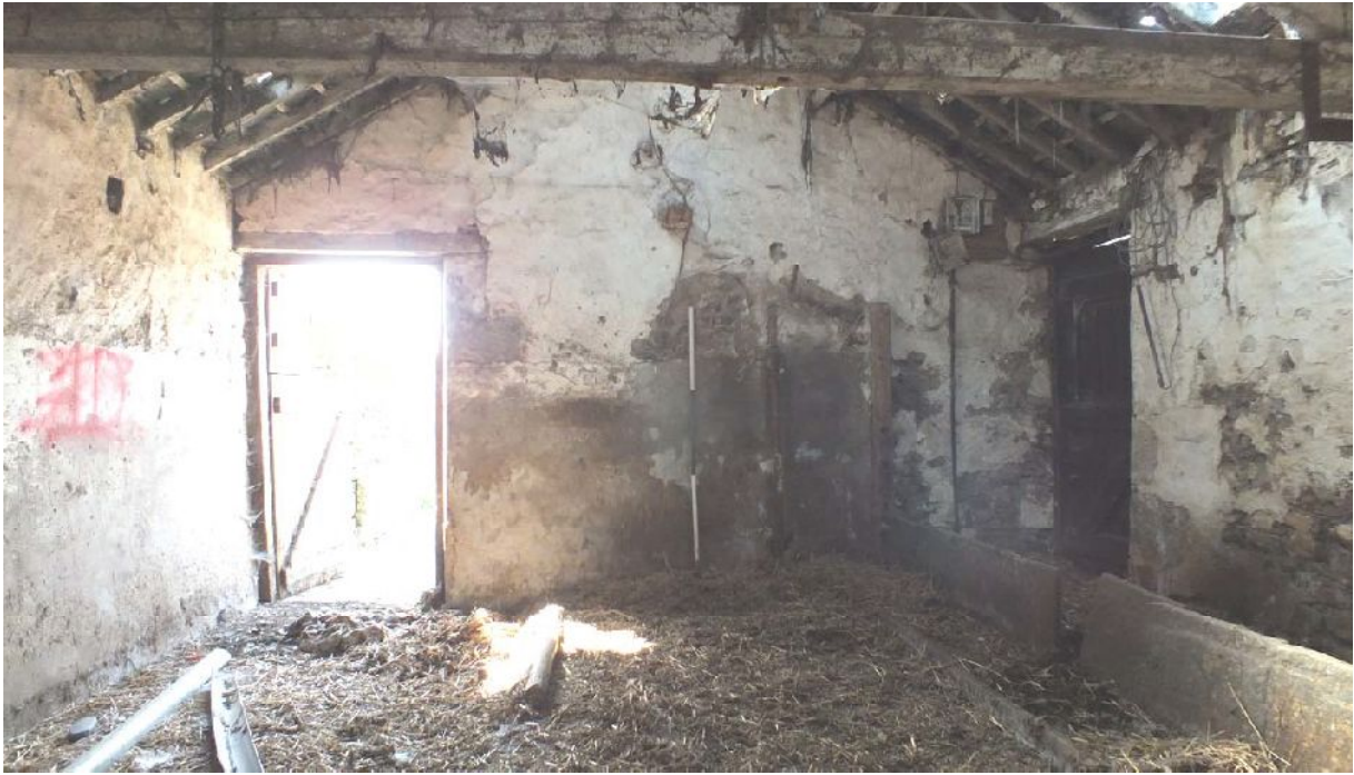
Plate 56: South-east elevation of Building C, from the north-west
