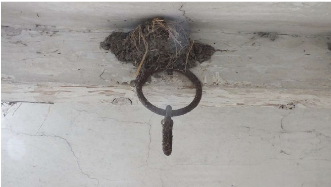
Plate 48: Loop in first floor Room 1 of Building B, from the north
