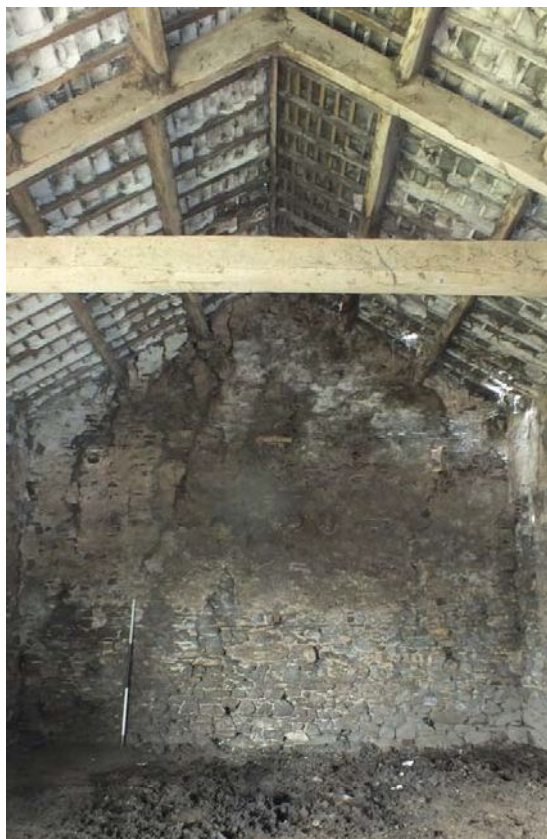
Plate 36: West elevation of upper floor of Building A, from the east
