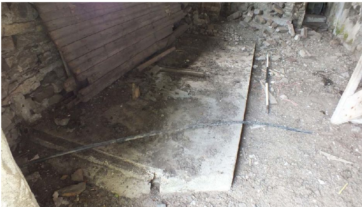
Plate 37: Floor of lower floor Room 1 of Building B, from the east
