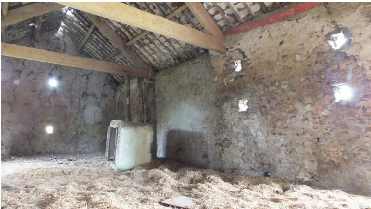
Plate 35: South elevation of upper floor of Building A, from the north-west
