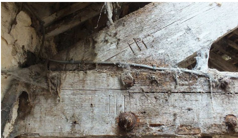
Plate 54: Carpenter's mark III in Building C, from the south-east
