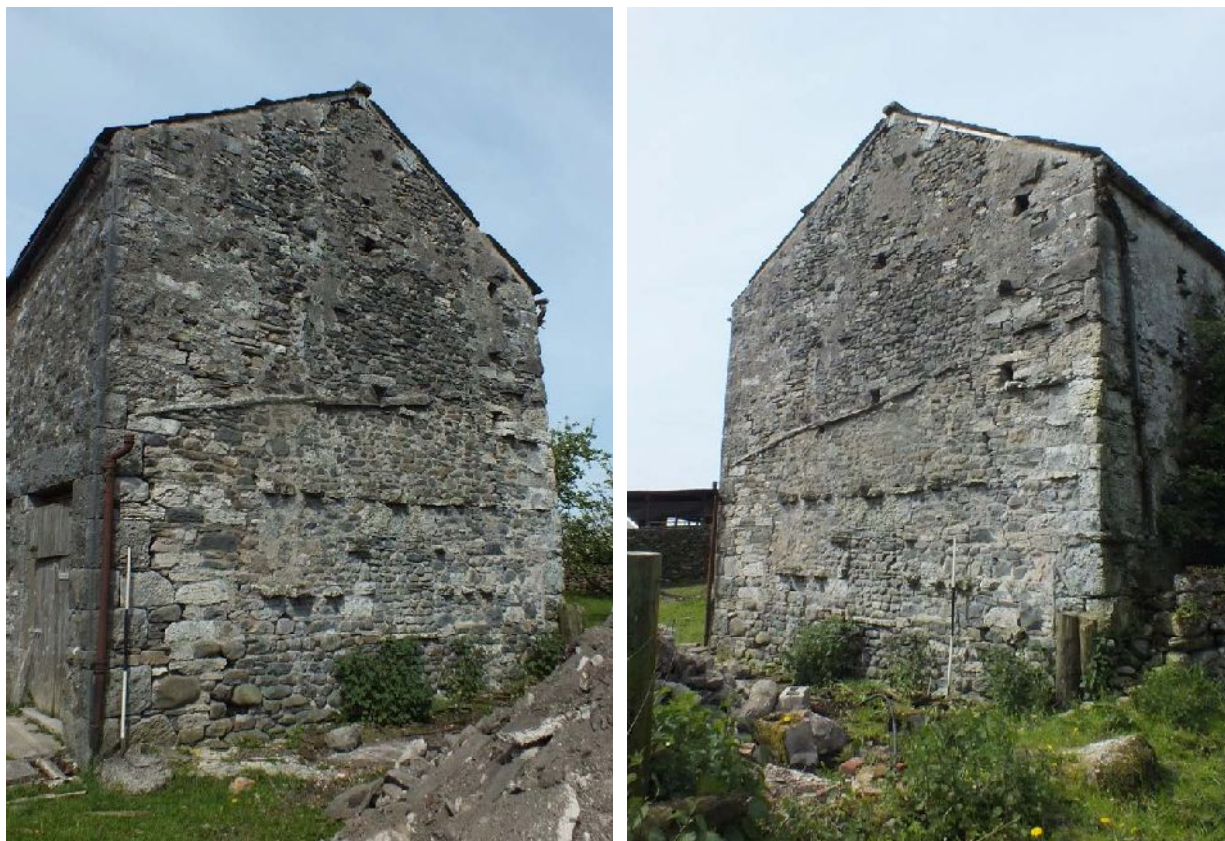
Plate 11 (left): East elevation of Building A, from the south-east
