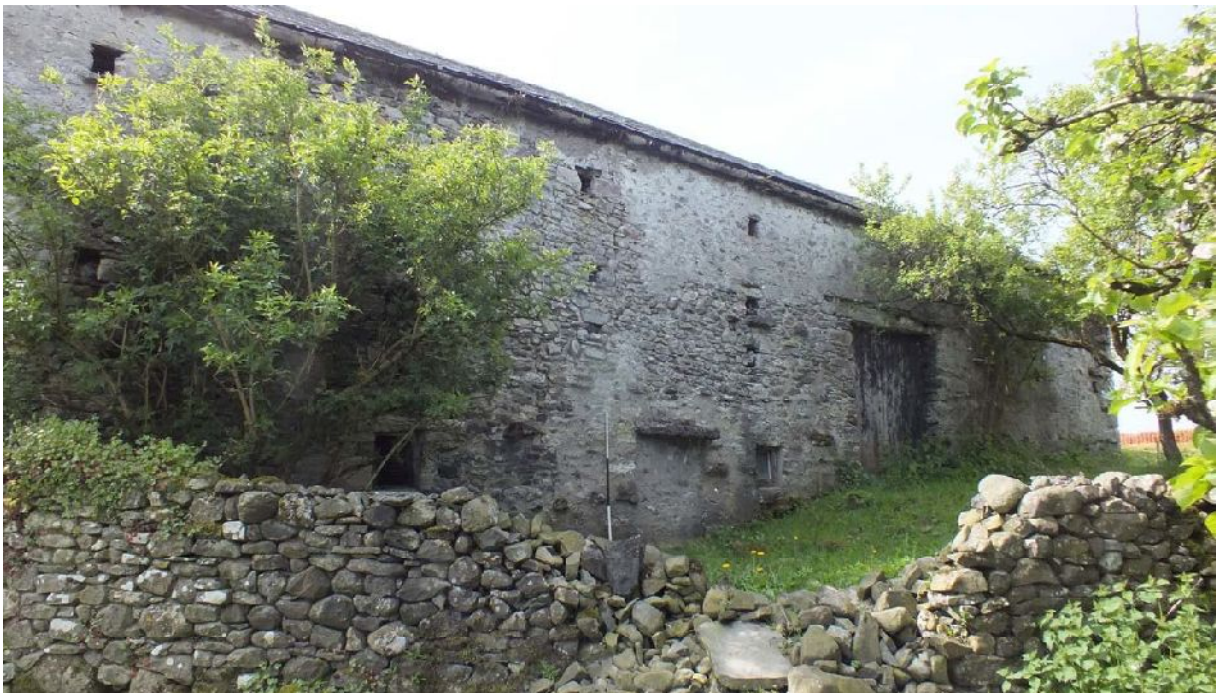
Plate 7: North elevation of Building A, from the north-west
