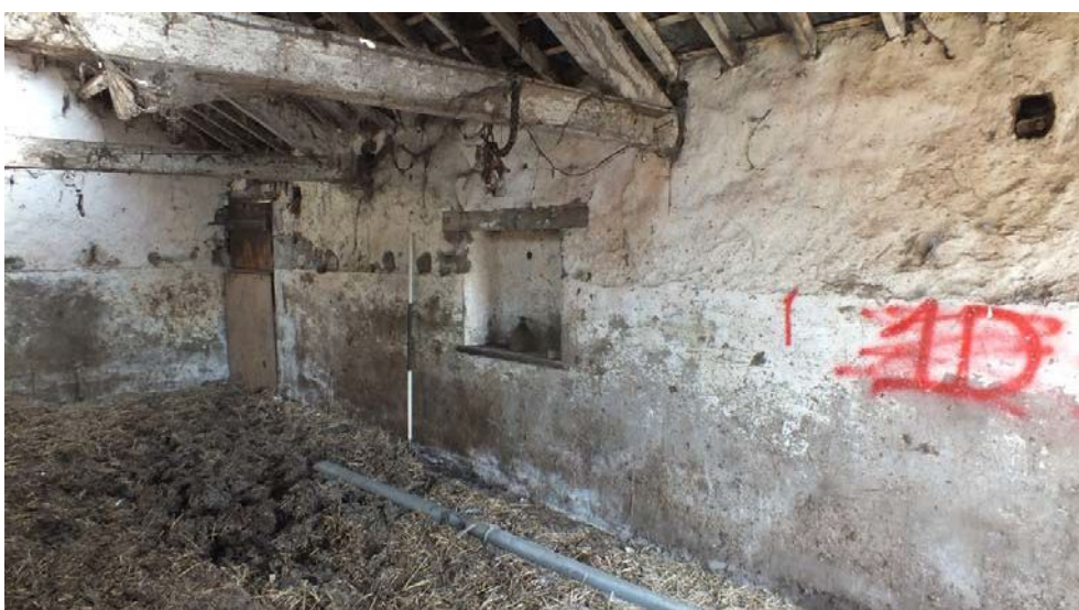
Plate 55: North-east elevation of Building C, from the south
