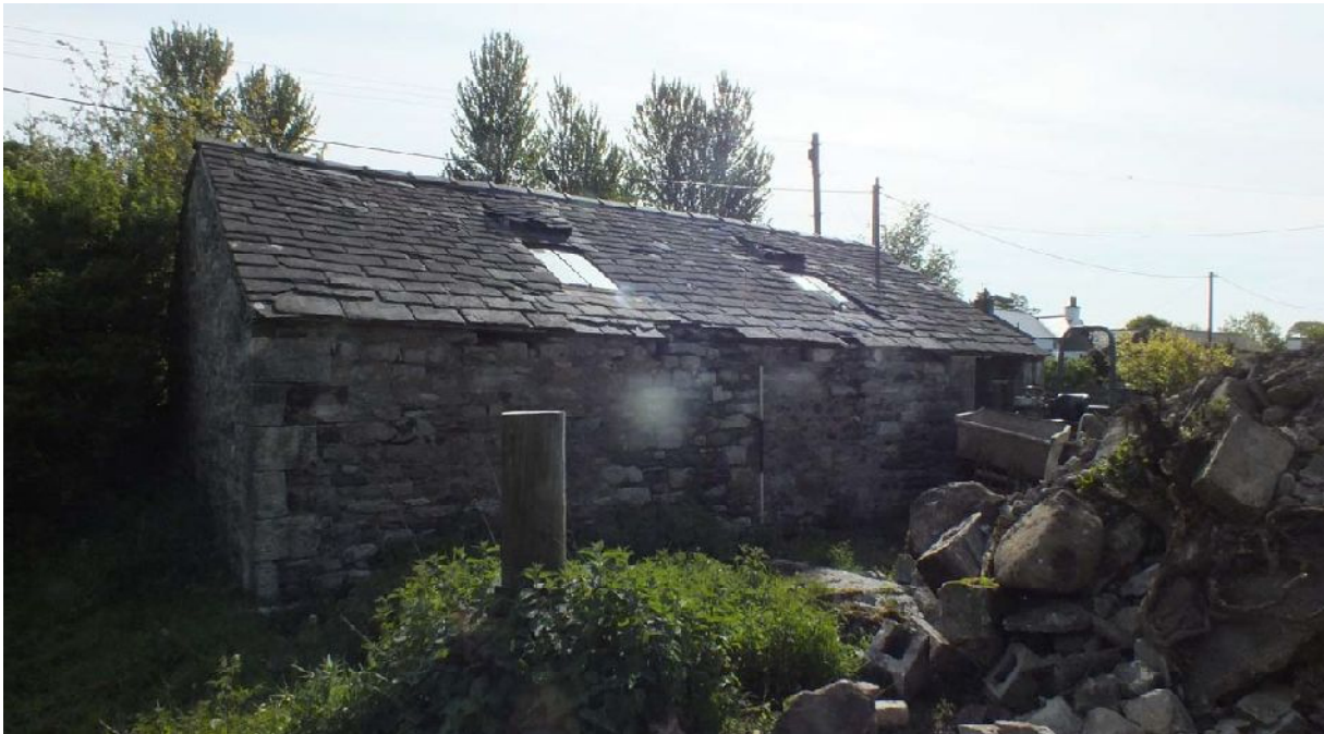
Plate 20: South-west external elevation of Building C, from the west
