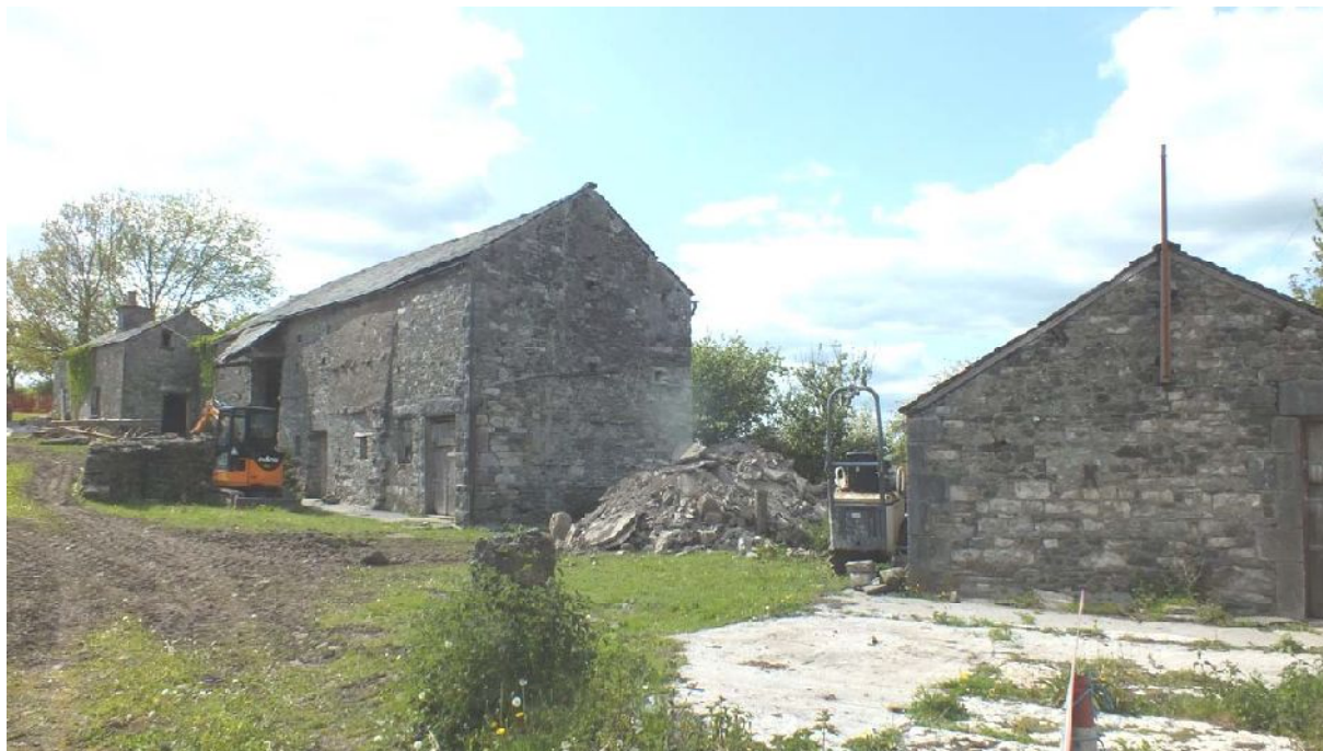
Plate 5: General view of the site from the south-east showing the relationship of the three buildings
