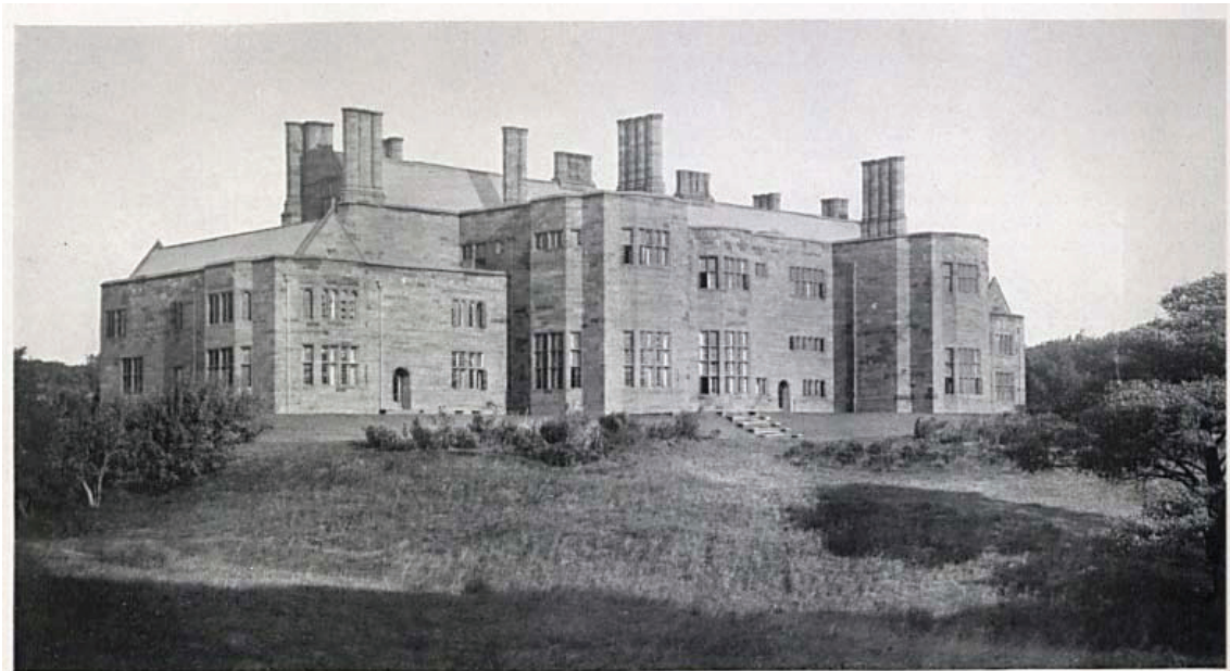
Plate 10: View of the terraces to the rear in 1921 (from Hussey 1921, 400)
