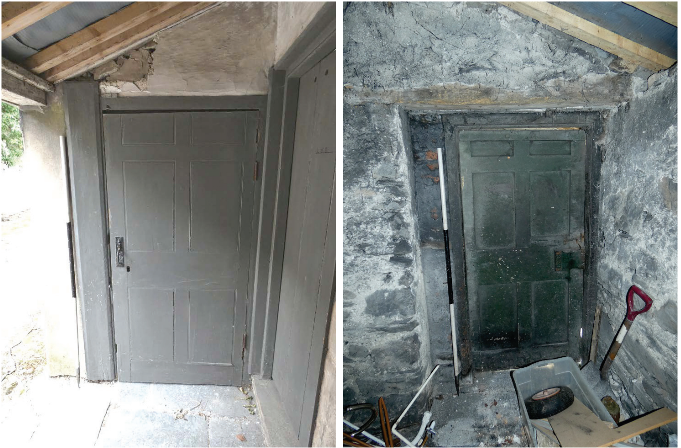
Plate 27 (left): Doorway to the south, Room G2, viewed from the north
