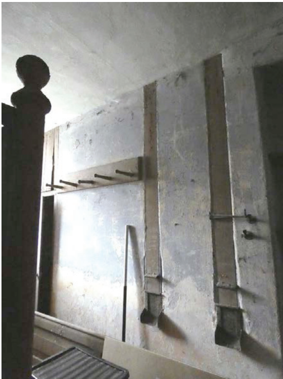
Plate 40 (left): Grain chutes built into the east wall of Room G6, viewed from the south-west
