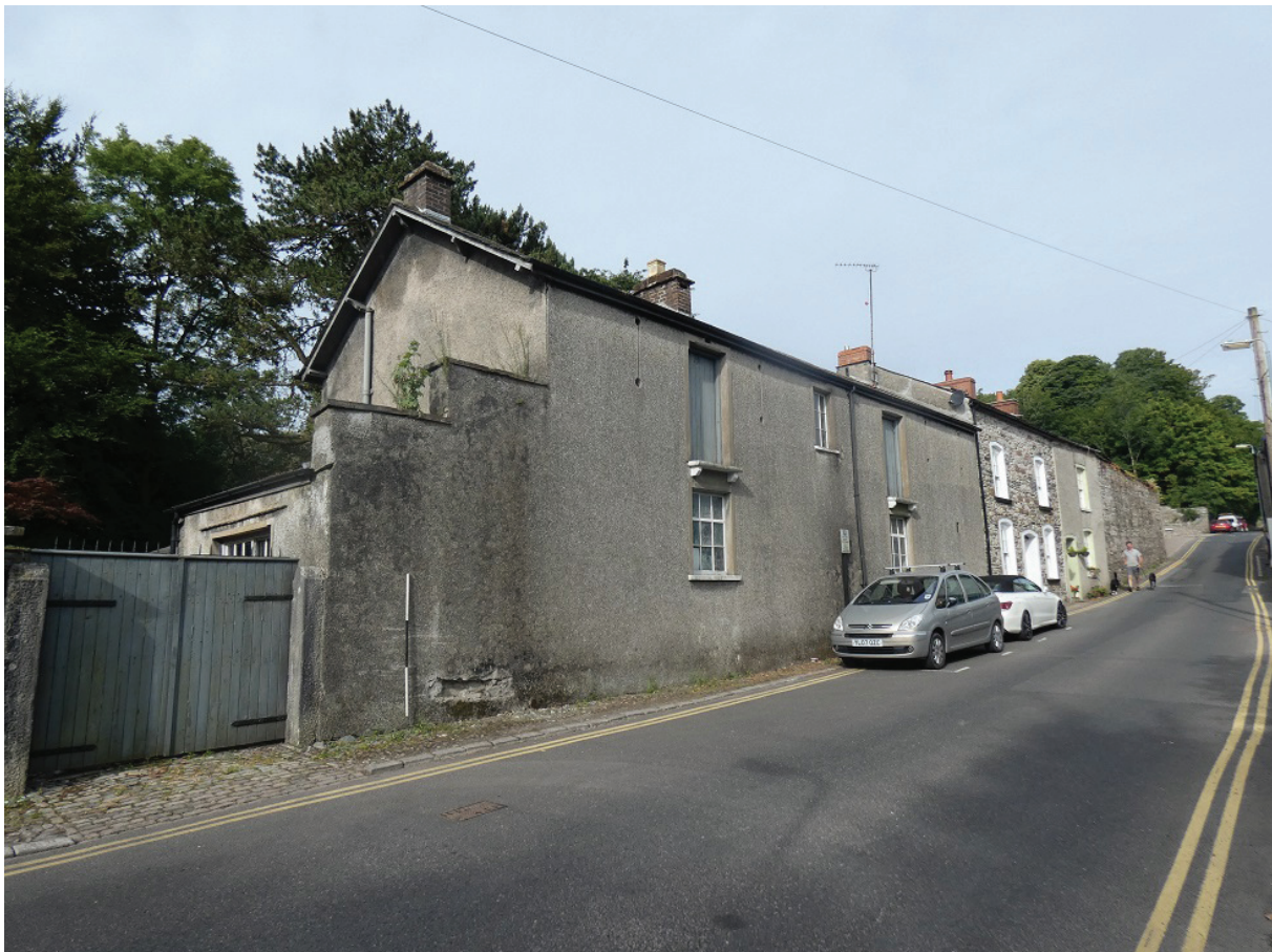
Plate 11: General view of the north external elevation, from the north-east
