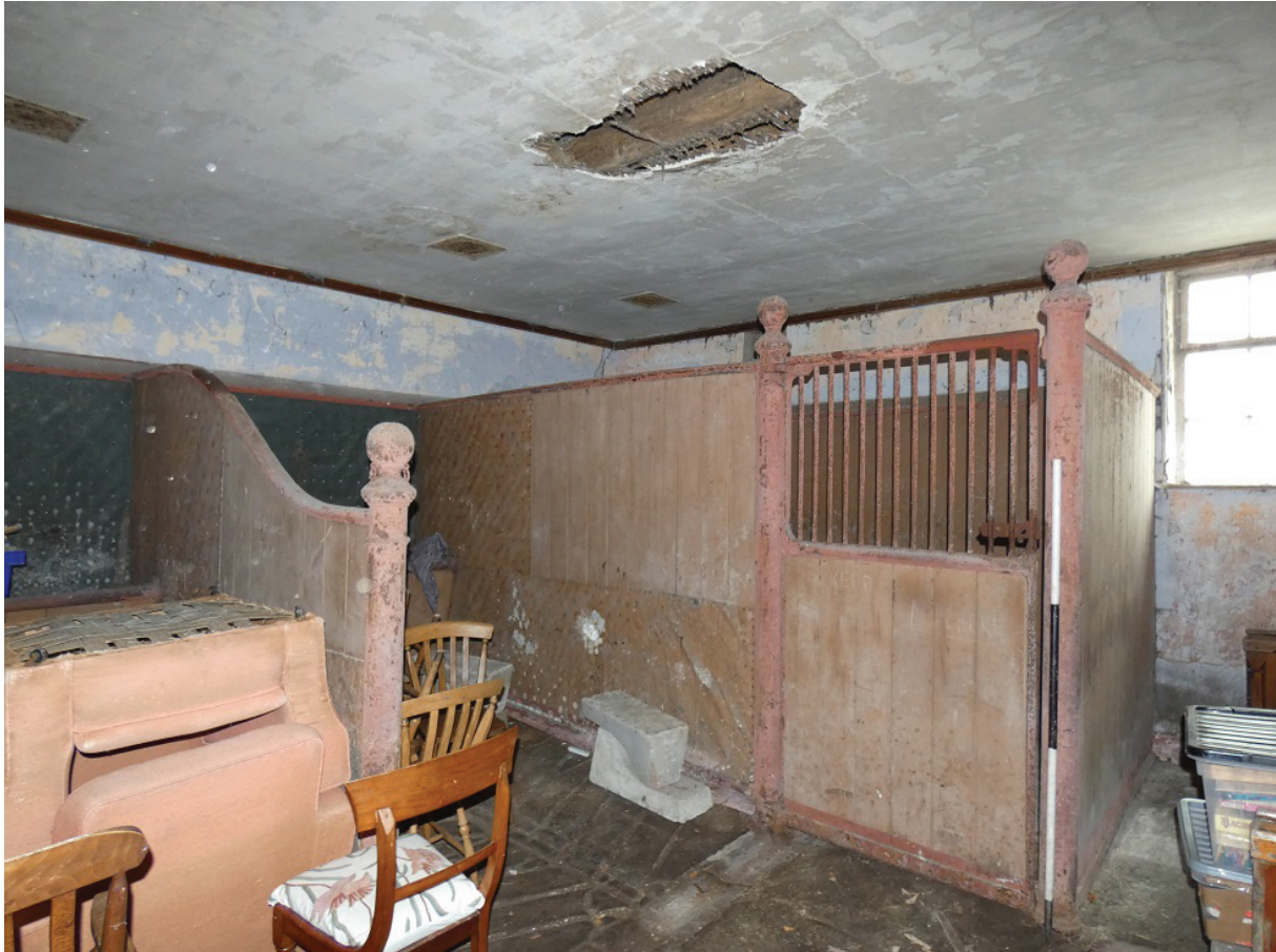
Plate 38: Stalls in Room G6, viewed from the south-east
