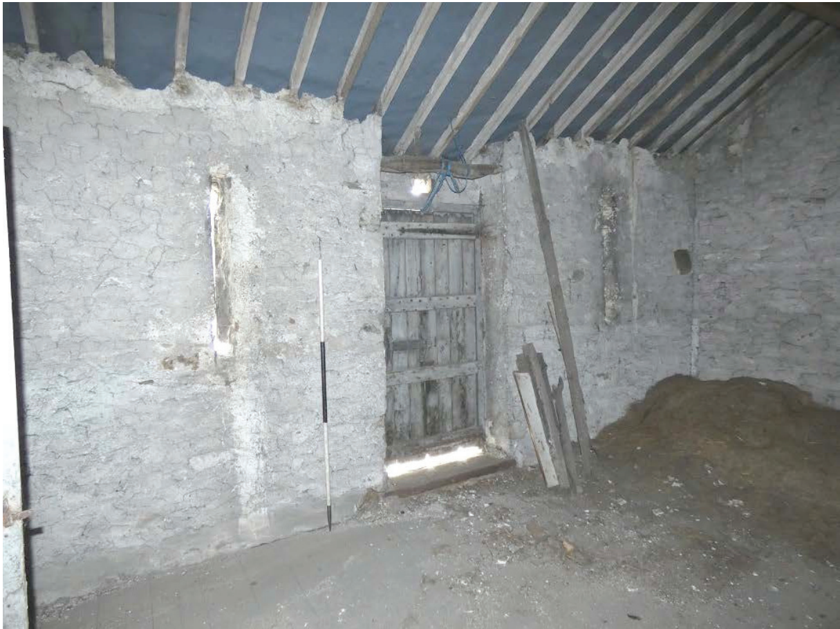
Plate 46: North elevation of Room F1, viewed from the south-west
