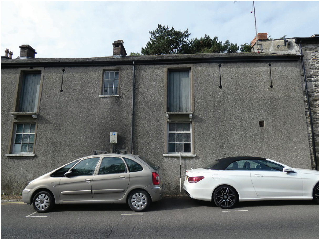
Plate 12: Detailed view of the north external elevation, from the north
