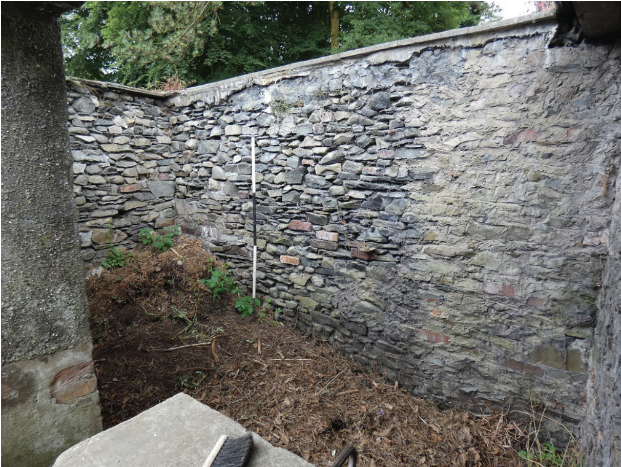
Plate 45: General view of Room G8, from the north-west
