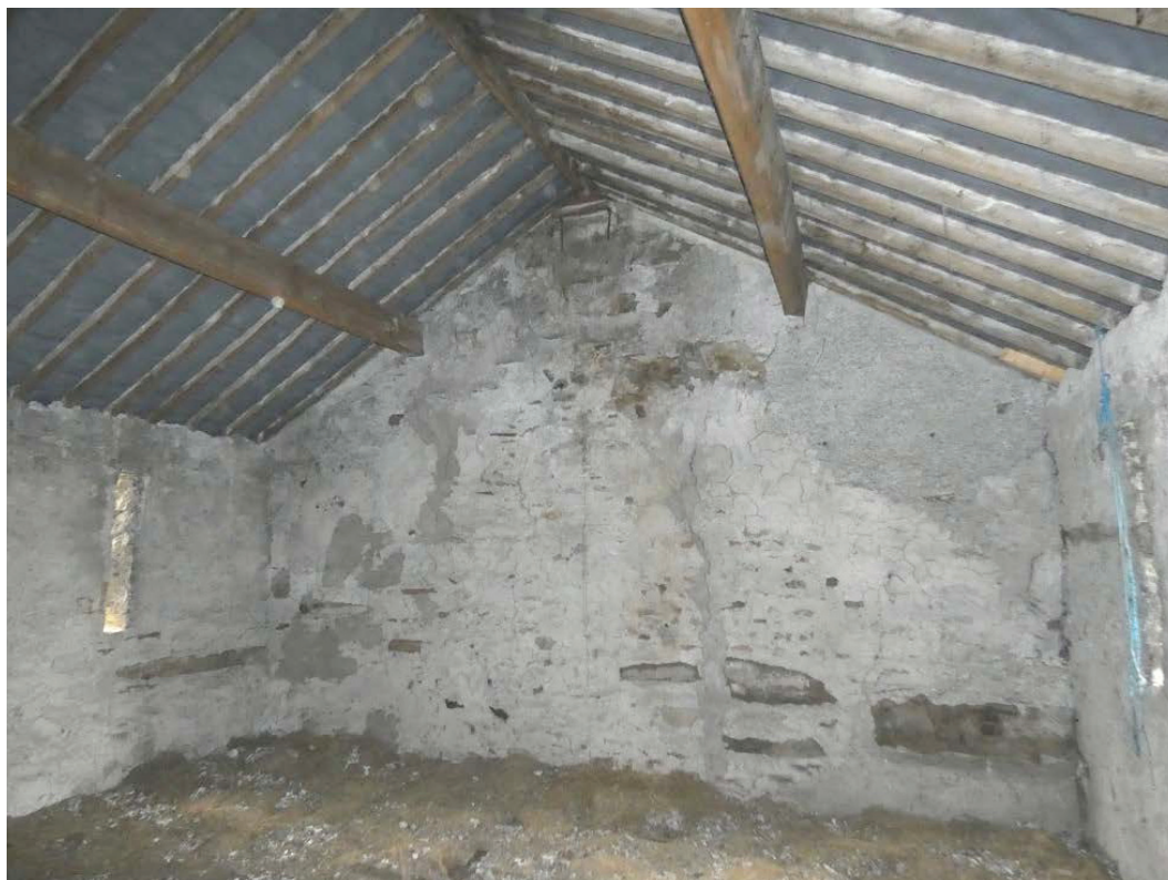
Plate 57: West elevation, Room F4, viewed from the east
