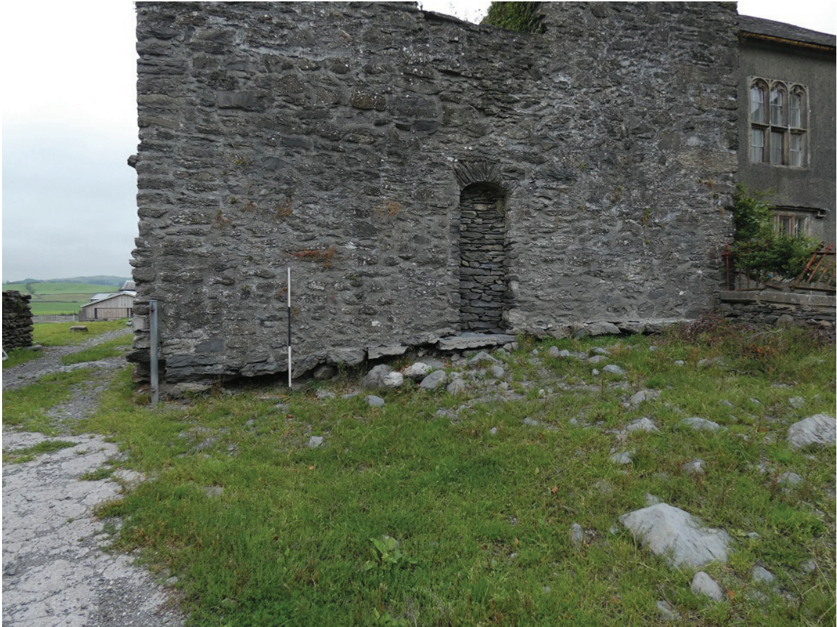
Plate 6: Detail of the site prior to excavation, showing the alcove and metal gatepost
