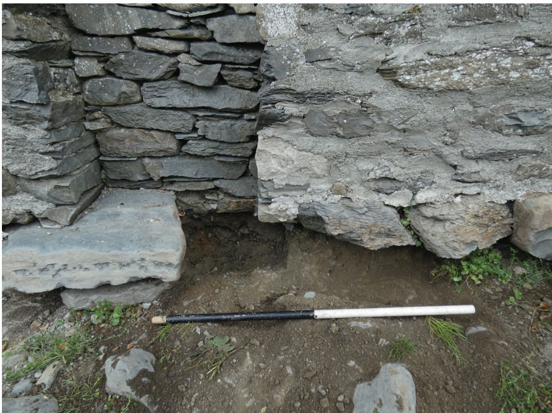
Plate 9: Excavation below the loose plinth stone on the south-east side of the alcove revealing deposit 103
